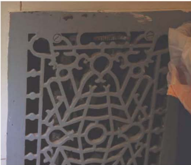
Air grate detail.
