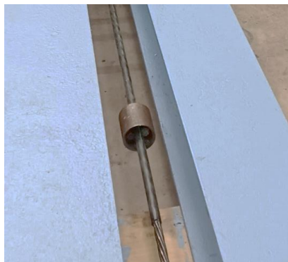
(c) Steel tension ring with strand fillers
