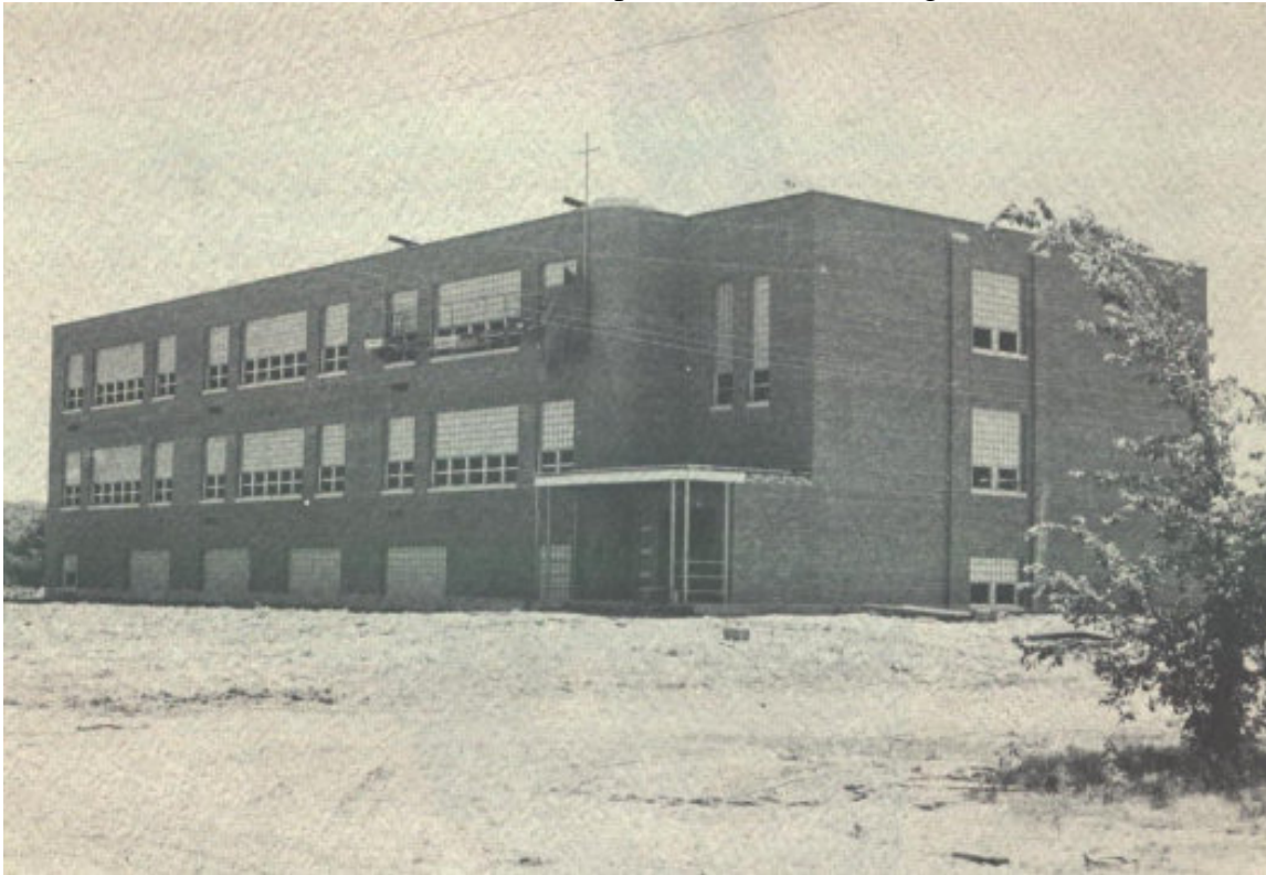
Illustration 8d. Completed School Building
