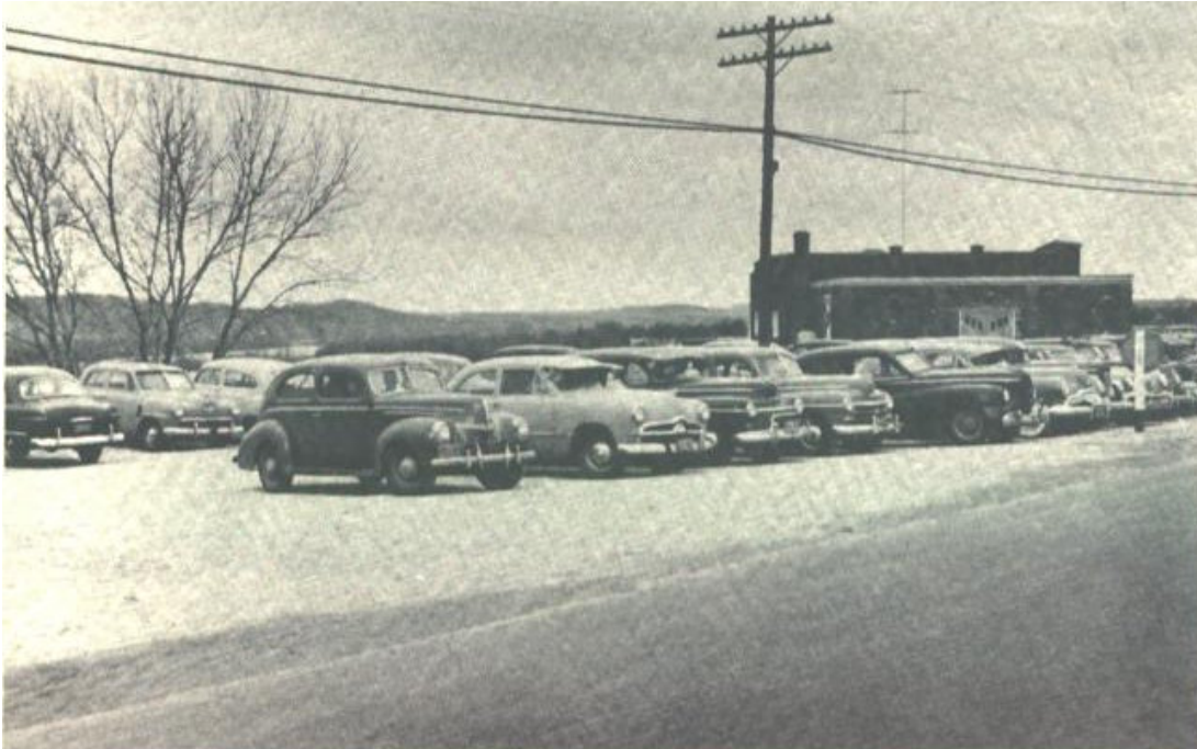
Source: St. Olaf Parish, "Dedication Souvenir of the Parish of St. Olaf" (parish document, Eau Claire, WI, September 26, 1954), 11.
