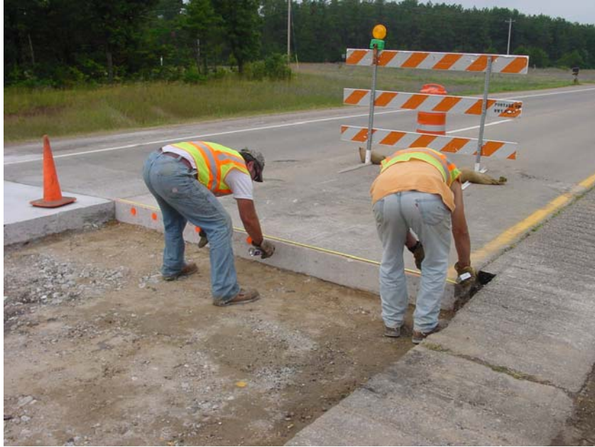
Figure 17. Marking out locations in the existing PCC for drilling.
