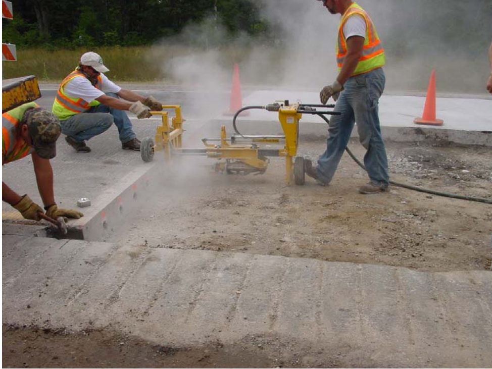
Figure 19. Drilling the existing PCC.
