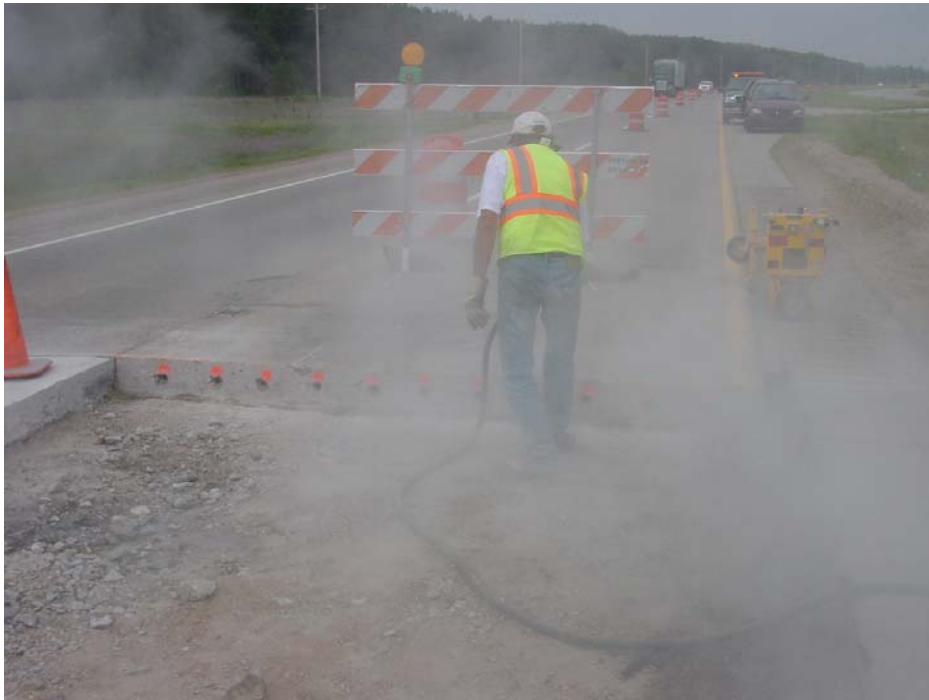
Figure 20. Cleaning drilling dust.
