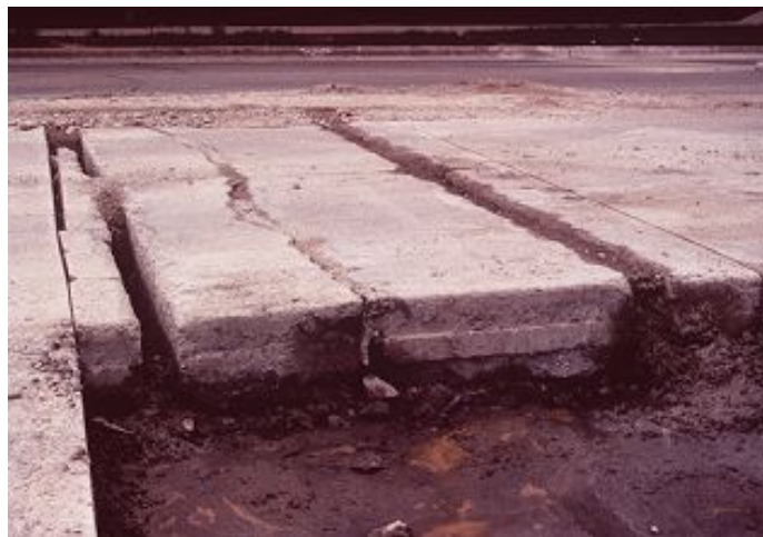
Figure 14. Partial-depth and full-depth saw cuts for CRCP. (10)
