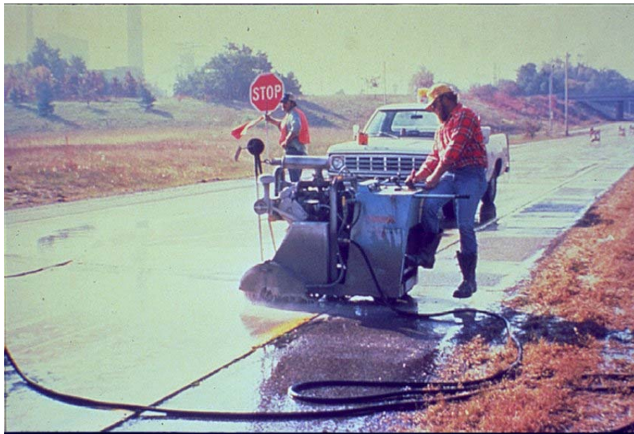
Figure 12. Sawing of full-depth repair transverse boundaries. (10)
