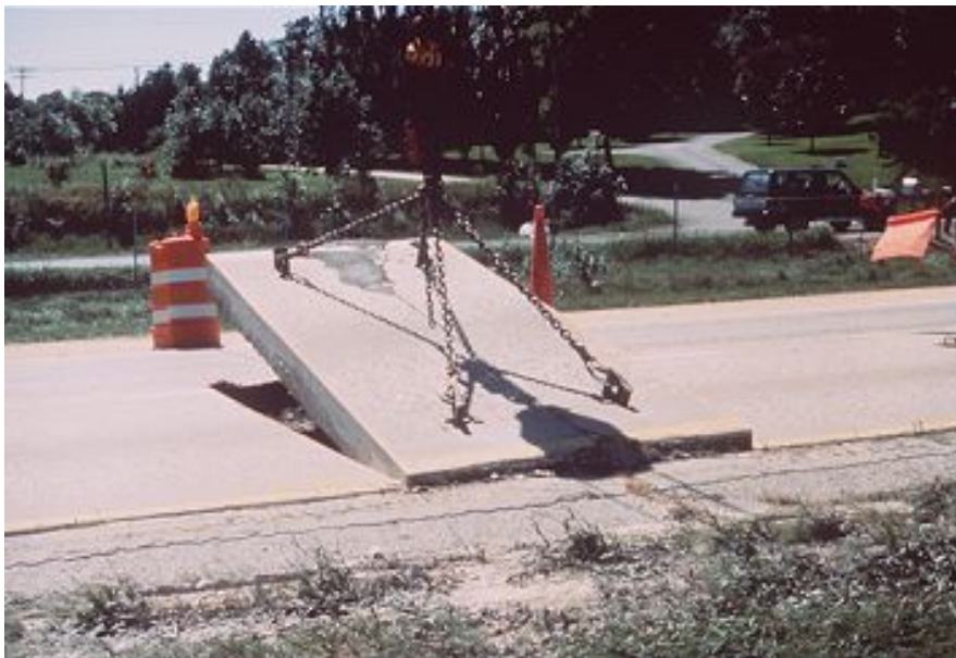
Figure 16. Lift-out operation chain for removing existing slab.
