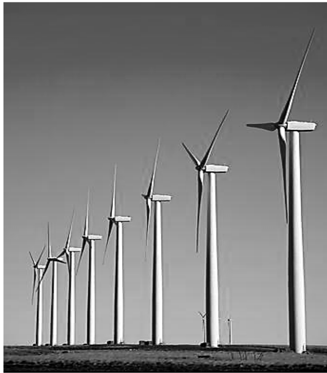
Figure 1.1 Big Horn Wind Farm at Bickelton, Washington
