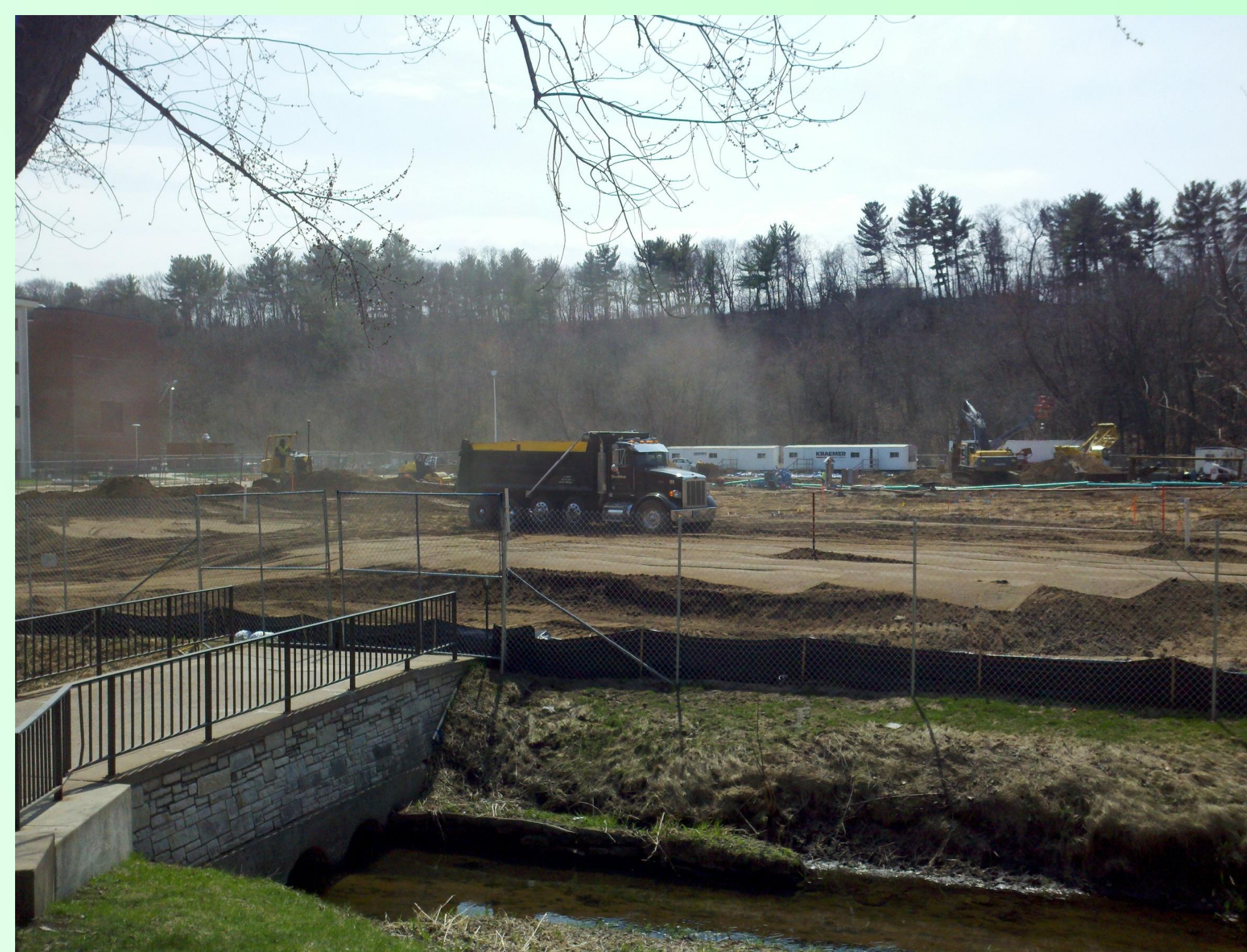
Student union construction; University-Wisconsin Eau Claire. Photo by Andrew Kleist.
