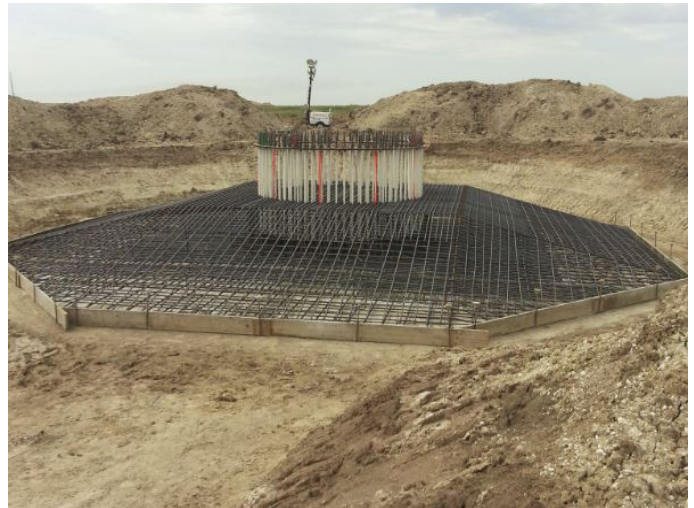
Fig. 2: WTG foundation during construction (© James Tinjum)
