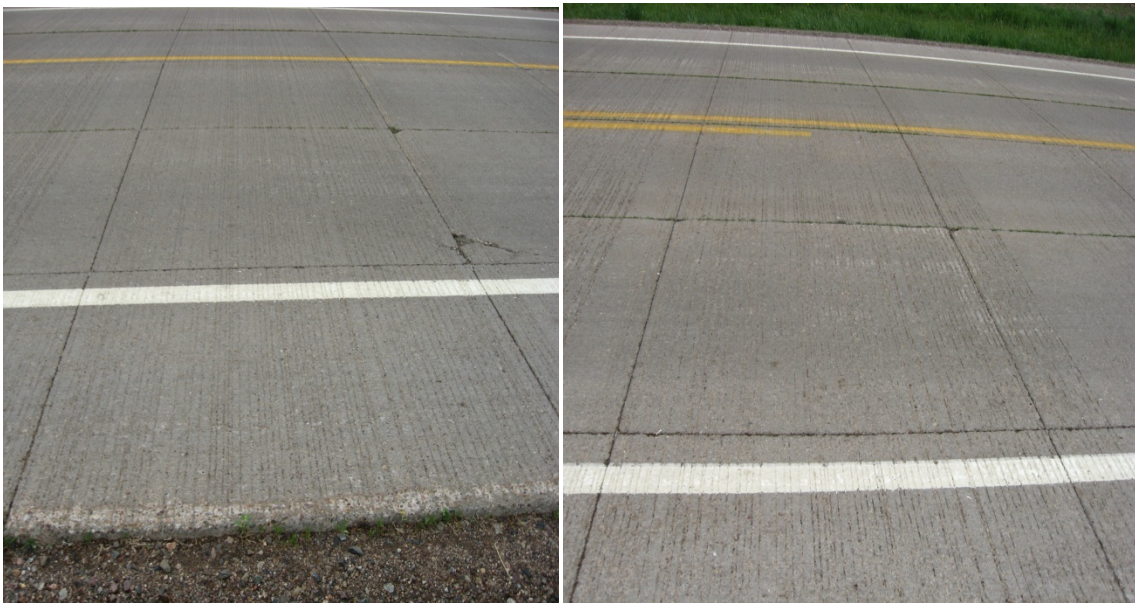
Figure 28. Condition of STH 97 (2008)
