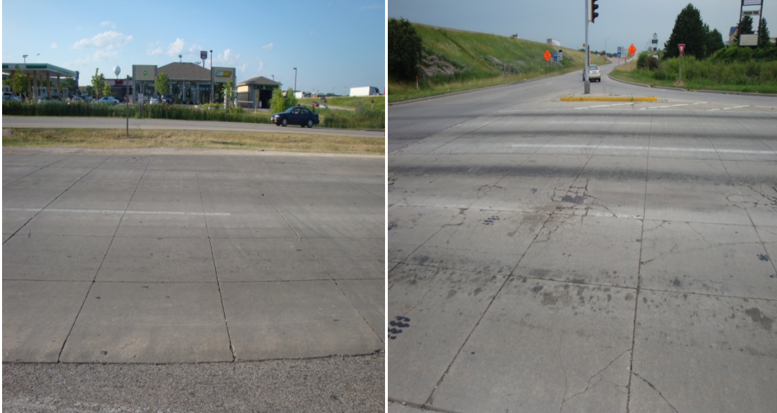
Figure 25. Condition of STH 50 (2009)
