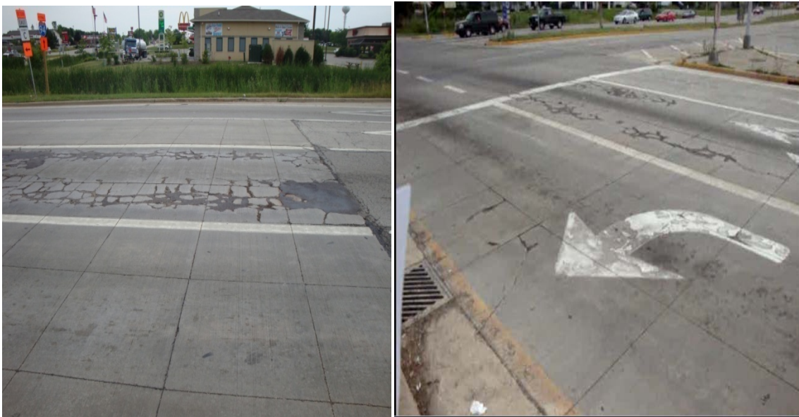
Figure 44. Localized Severe Distress at the Entrance (left) and Exit (right) End of IH94/USH50 Ramp
