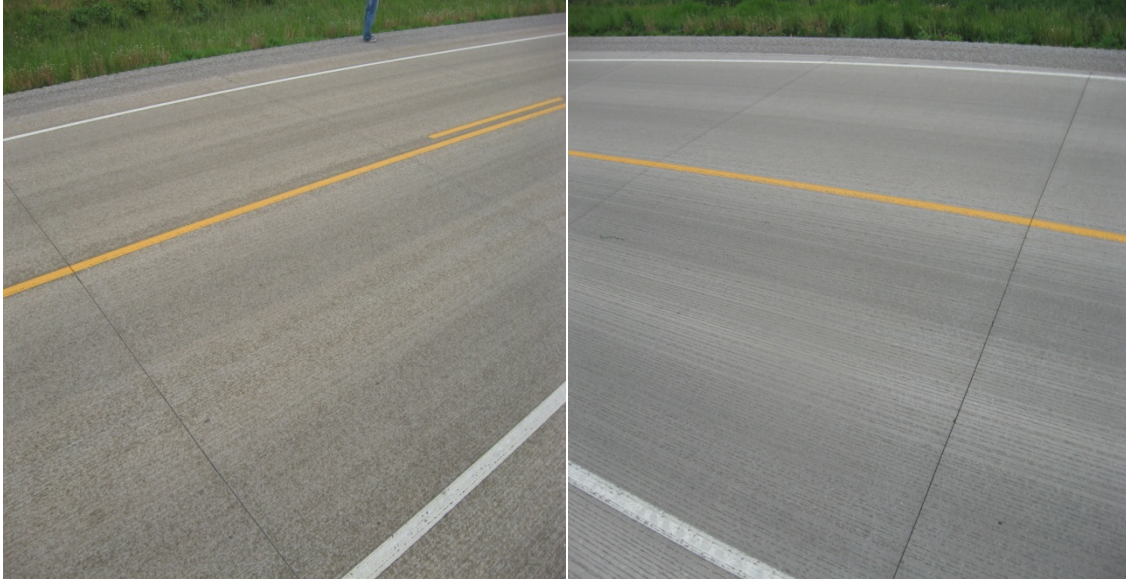
Figure 16. Condition of CTH “A” (2008)
