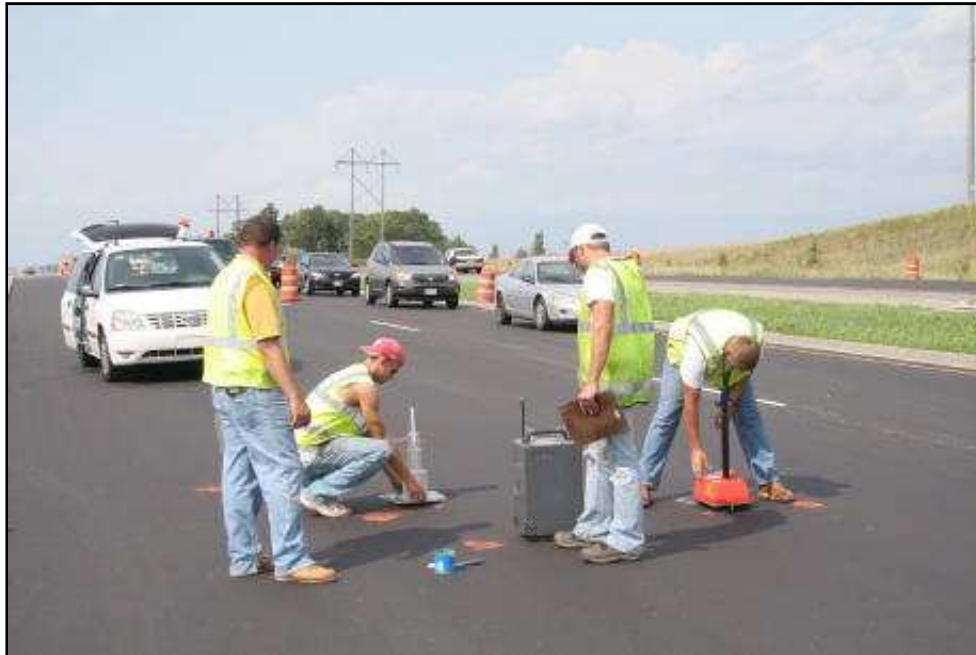
Figure 3.1 Testing for Permeability and Density (USH 41 Fond du Lac County)
