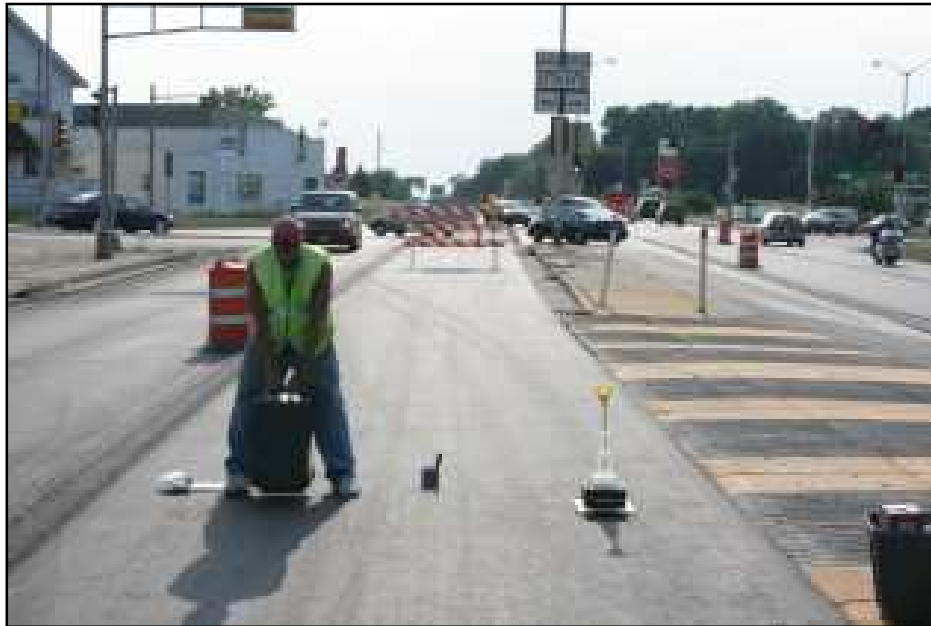
Figure 3.2 Permeability Testing (STH 60 Washington County)
