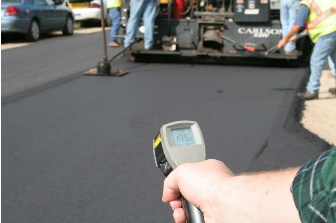
Figure 6.6 Warm Mix Temperature Reading behind Paver
