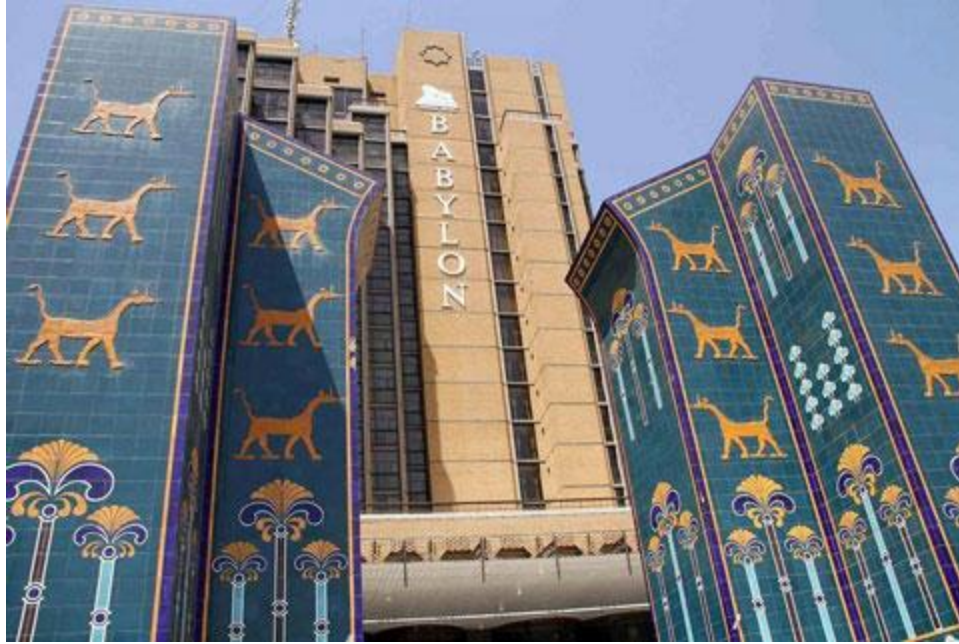
Figure 3.4. Stylized Ishtar gate entrance Baghdad. Image from Building the Non-Aligned Babel: Babylon Hotel in Baghdad and Mobile Design in the Global Cold War (Kulić 2015: Fig. 2) ( https://journals.openedition.org/abe/docannexe/image/924/img-2.jpg ).
