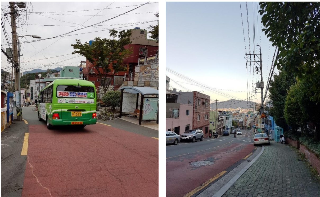
Figure 13 Narrow road conditions of Sanbokdoro for traffic
