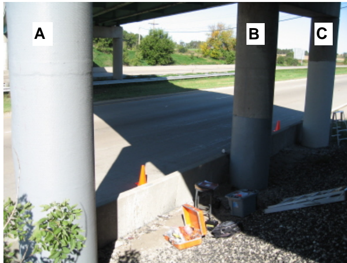
Figure 4.11: Tested columns in the Bridge B-53-71 (Northbound).
