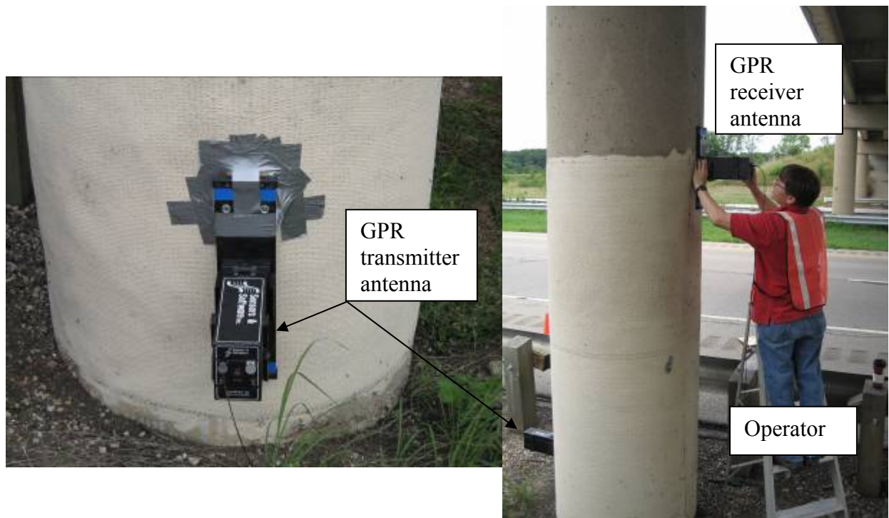
Figure 4.21: GPR testing setup and data collection on a fiberglass wrapped column.
