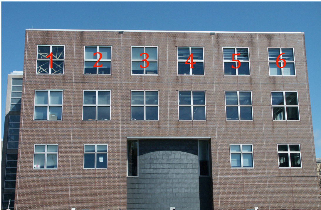
Fig. 3.5: The west façade of the building. Windows 1, 2 and 3 are original windows. Windows 4, 5, and 6 are subdivided windows.
