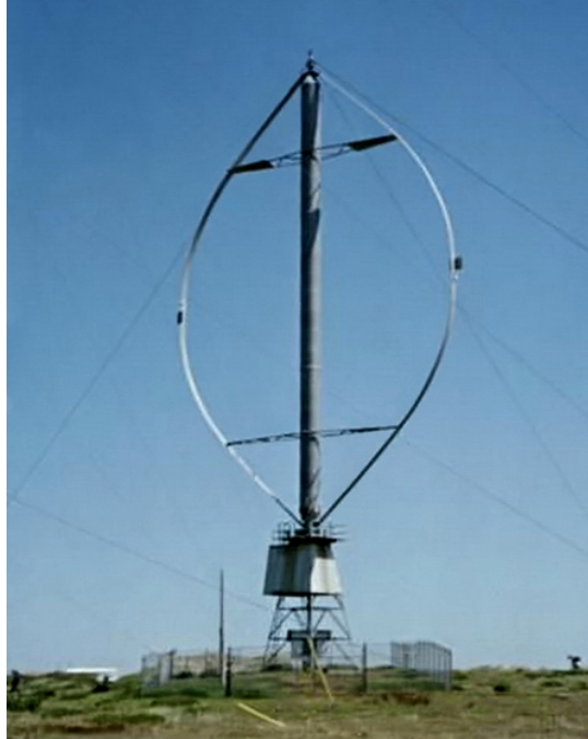
Fig. 1.2 A Darrieus Type Vertical Axis Wind Turbine [6]
