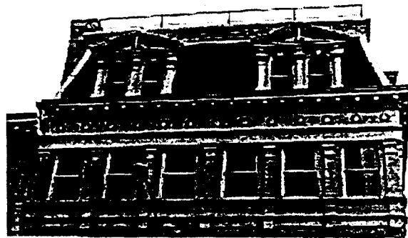
Figure 8: The two story addition was considered important to the overall shape of the Curry-Pierce Building.
