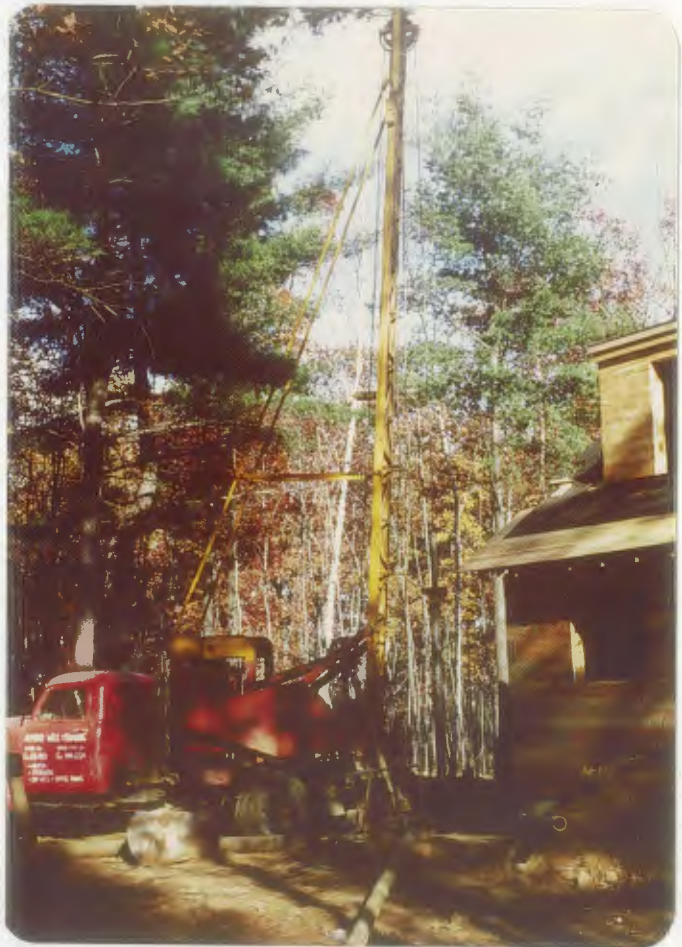
Figure 7. Cable drilling rig used at the Porter road site.
