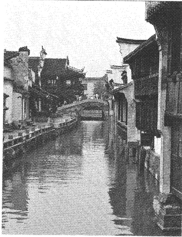
Figure 4.14: The firewalls between the buildings in Nanxun. Source: Photograph by Yan Zhang, 2004.
