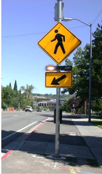
Figure 7: A rectangular-shaped rapid flash LED beacon system (Systems, 2009-2013)
