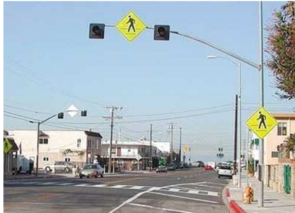
Figure 6: Overhead pedestrian sign (Pang, 2010)
