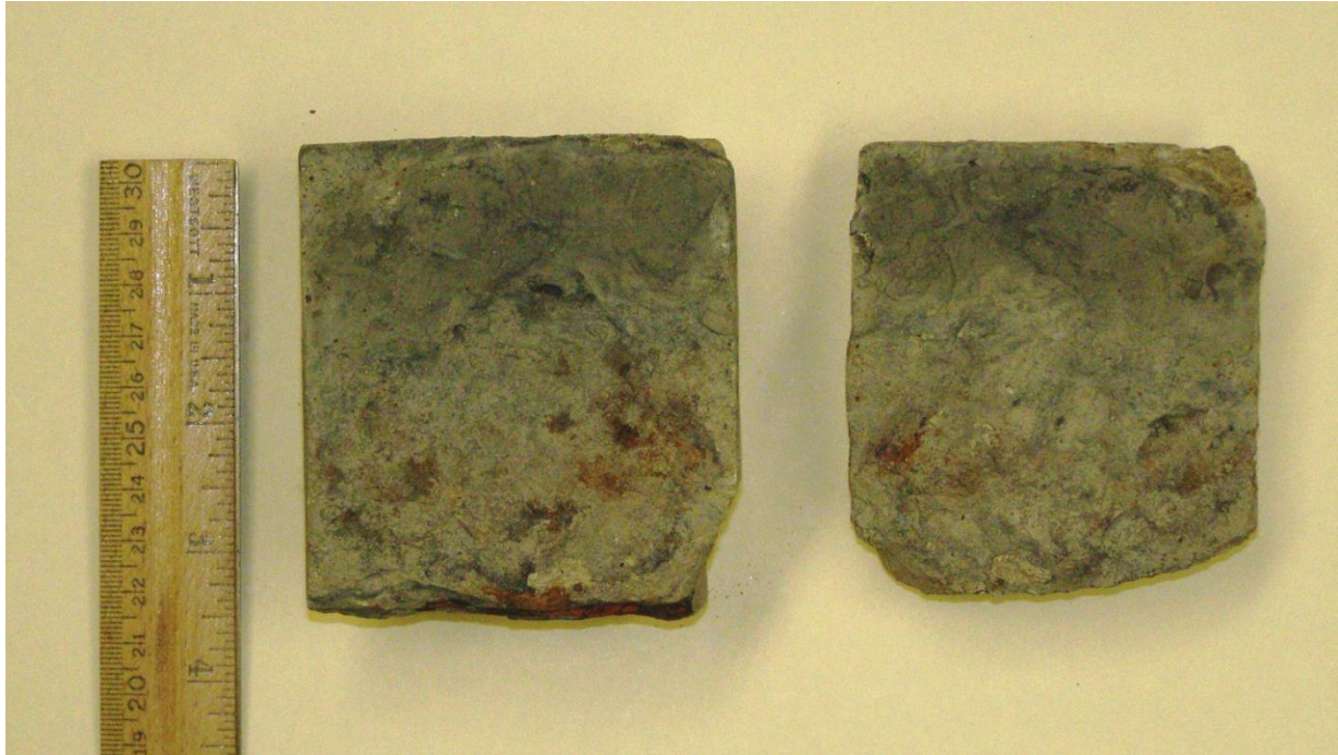
Figure 4.3 Evidence of carbon dioxide penetration through cracks in bridge B-13-0337.
