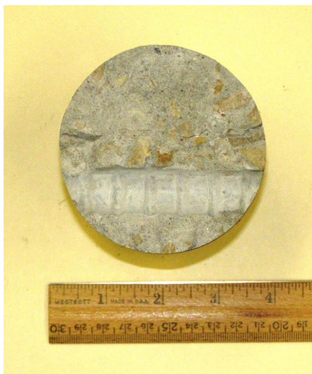
Figure 4.6 Bar markings (clean) on the bottom of a core extracted from bridge B-14-0034.
