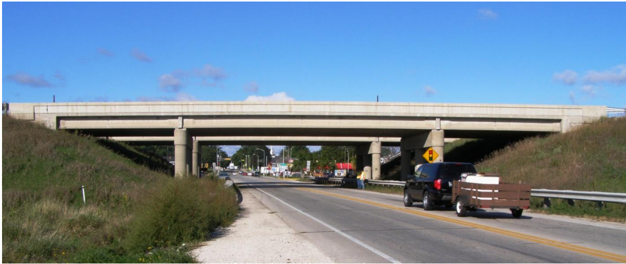
Figure 3.6 Overall view of bridge B-13-0034.
