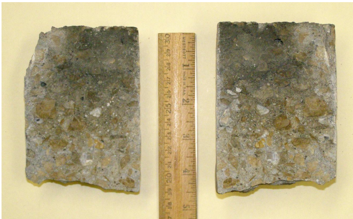
Figure 4.5 Evidence of carbon dioxide penetration through cracks in bridge B-14-0034.
