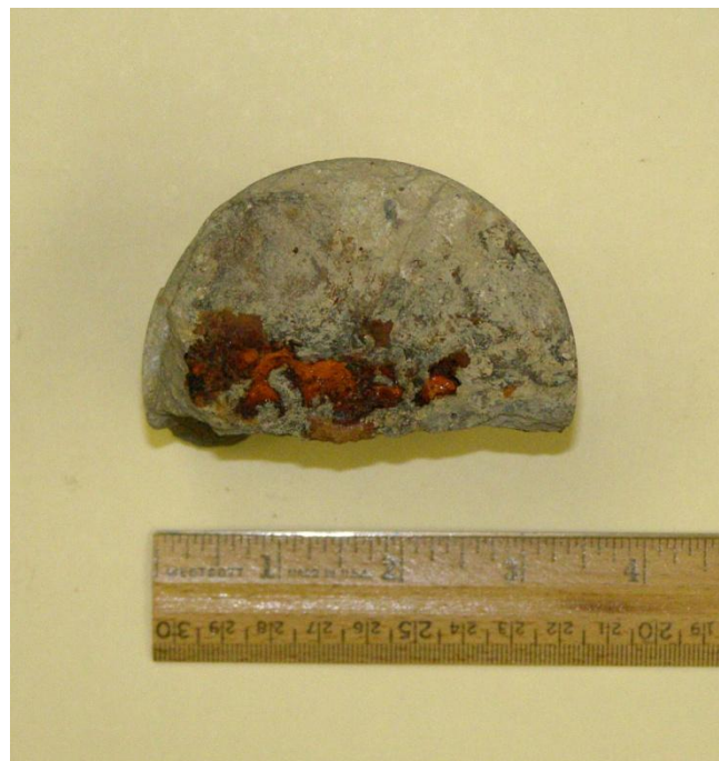
Figure 4.4 Rust stains on the bottom of a core extracted from B-13-0337.
