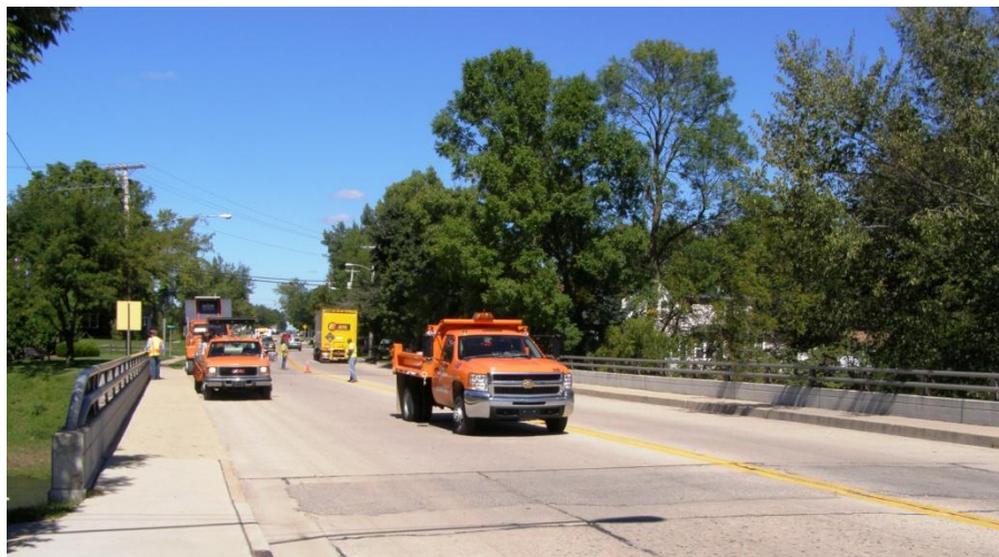
Figure 3.2 Overall view of bridge B-13-0337.
