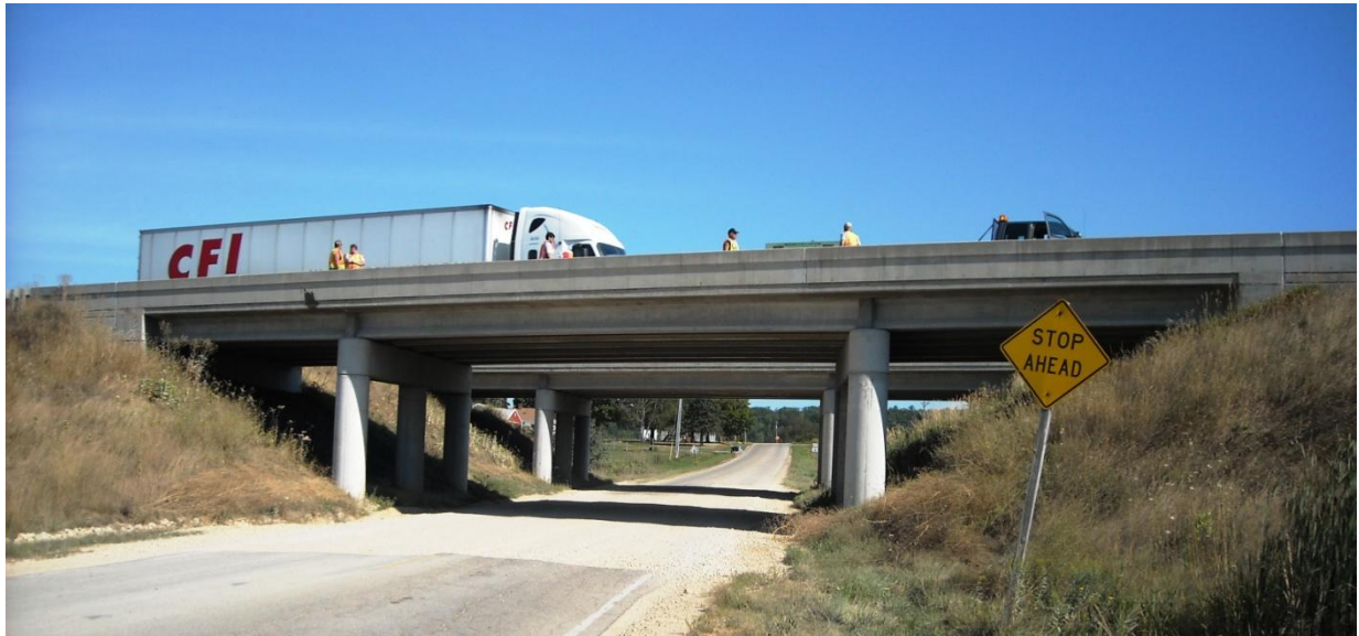
Figure 3.9 Overall view of bridge B-58-0080.
