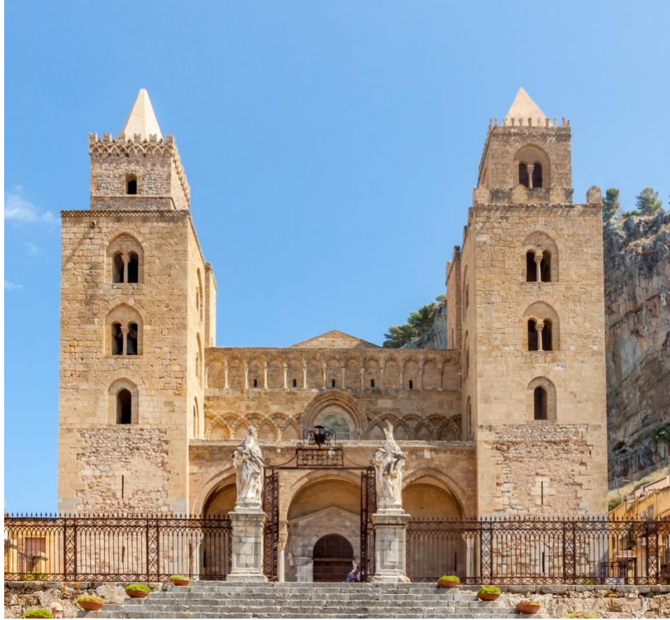
[Figure 4.4] This photograph shows the western entrance of the Cathedral of Cefalù in Cefalù, Sicily. Image accessed via Wikimedia Commons
