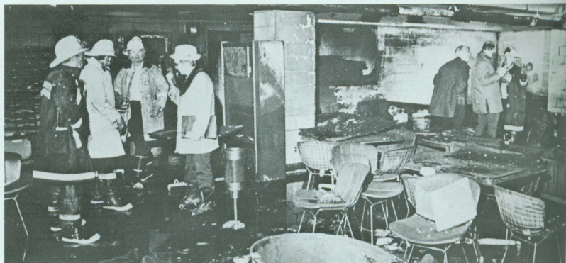
Fire inspectors survey damages in the Medical Student Lounge.
