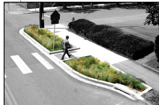
Green portion in extended bump-out used for stormwater management Seattle, Washington
