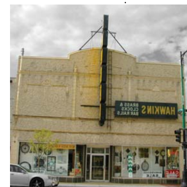
Corner bump-out intervention
