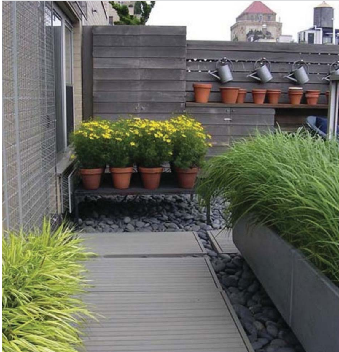
Roof Treatment with Wooden Pathways, Gravel Base Layer and Planters
