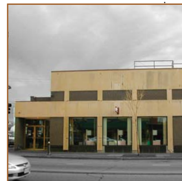
Corner bump-out intervention
