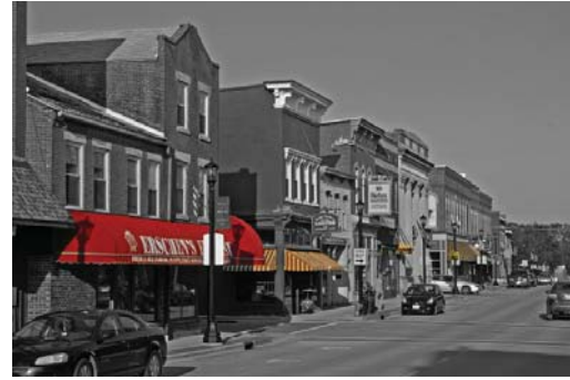
Regulation on awnings to achieve continuity in street facade Main Street, Platteville, Wisconsin
