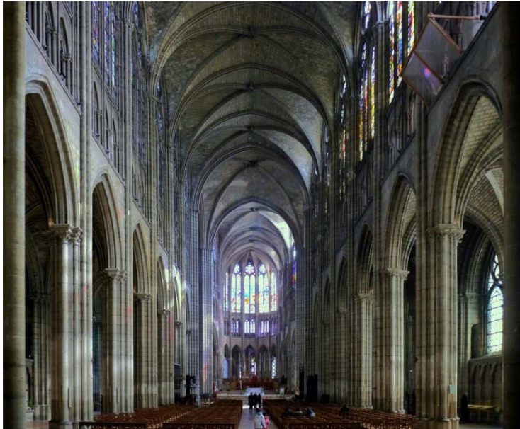
Figure 13 Rib-vaulted Nave of St. Denis looking toward the apse "Travel to Eat"
