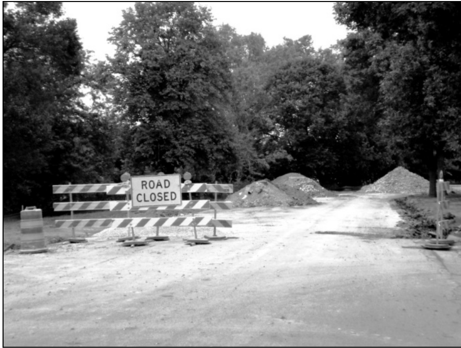
Photo 1 - McCormick Garden and pavement removal
