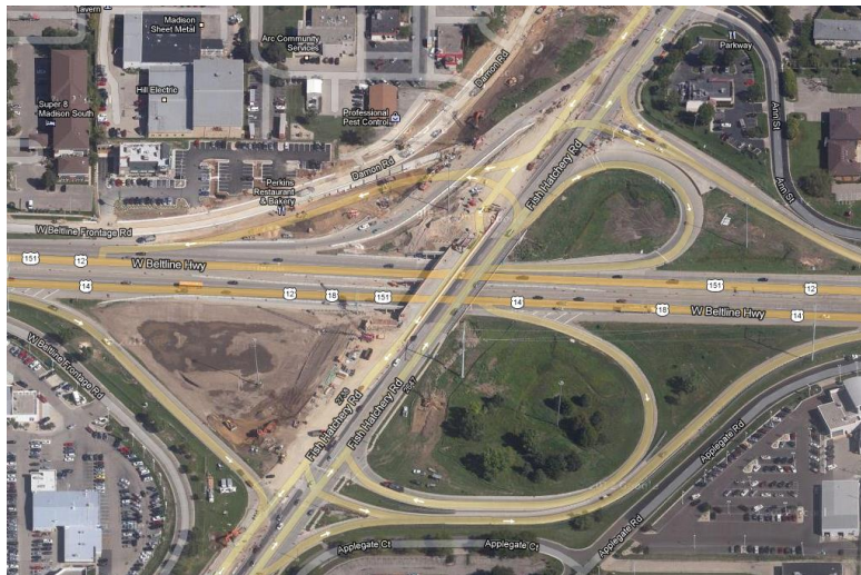
Figure 5.1 Image of Fish Hatchery Construction
