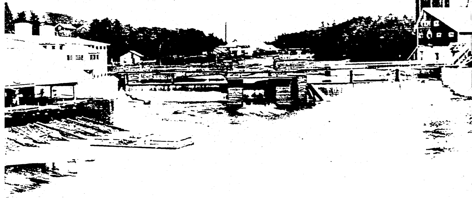
Eau Claire Lumber Company sawmill on north bank of Eau Claire River was located about 100 meters east of Dewey Street bridge. Building at immediate left is rafting shed where lumber cribs were assembled. Cribs slid down ways, and two cribs apparently have just hit water. Smoke stack looms farther up river, site of second dam and water powered shingle mill for same company. Third stack represents planing mill. At right, flour mill. Below, photo of same sawmill taken in 1873, shows mill had already been converted to steam. At right, probably original flour mill on this site. Compare above. Both probably operated off water turbines.
