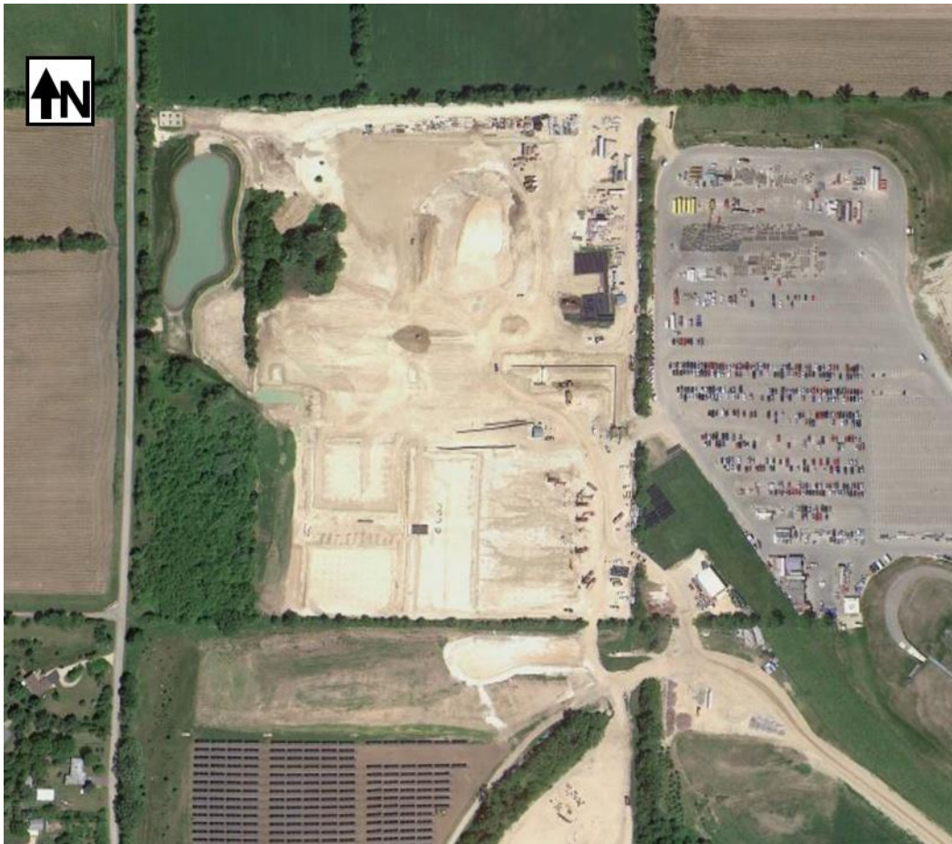
Figure 19: Aerial image of Borefield #4 obtained from Google Earth, dated June, 2014. The borefield is bordered to the east by Epic's North Parking Lot, and to the south by Borefield #3, which is covered by photovoltaic solar arrays in the image. The dimensions of the field are approximately 400-m (1300 ft) length by 250-m (820 ft) width.
