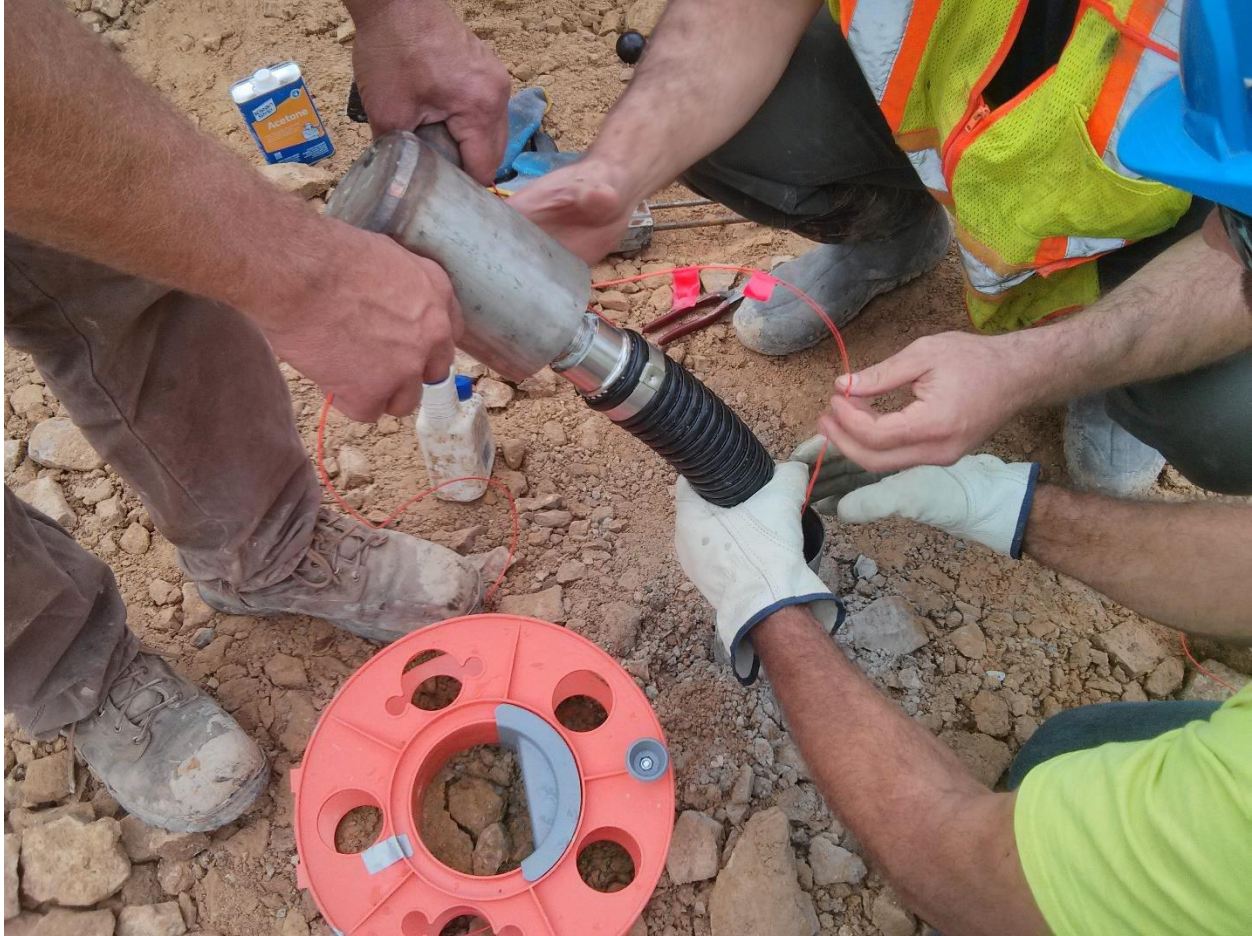
Figure 36: Stringing fiber through coaxial wellhead before permanently fusing to the GHE.
