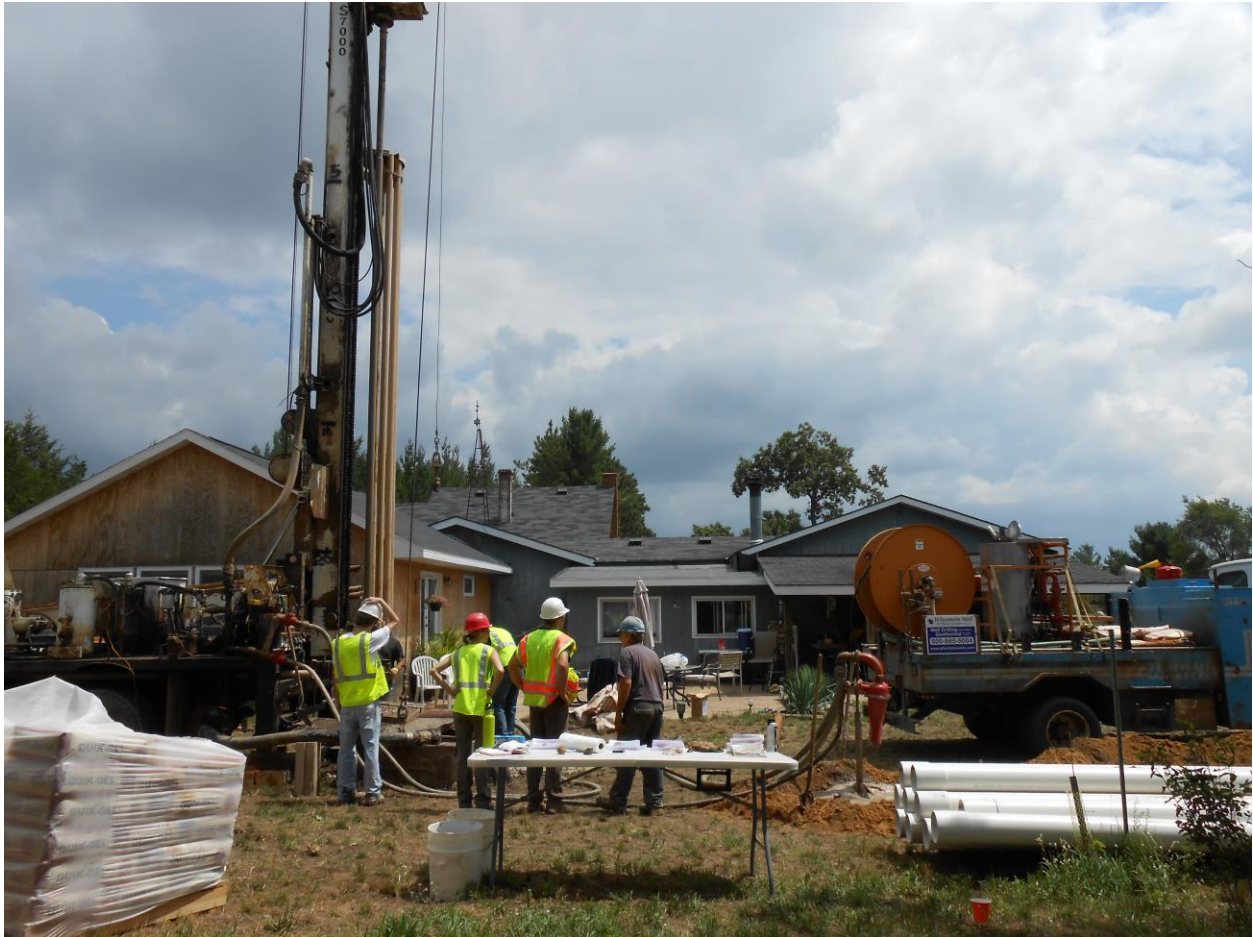
Figure 41: Photo of the drilling of the first GHE at the Grand Marsh residence (courtesy of Lauren Meyer).
