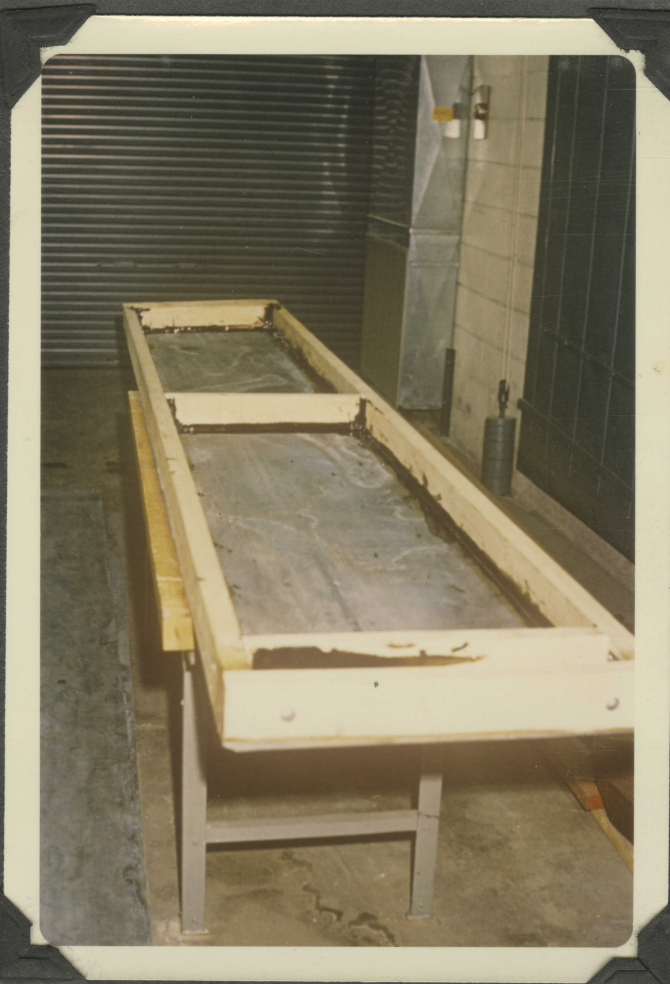
Figure 7. Basic construction of pontoon body showing pits for floatation and false ends. Sheeting is 18 ga. galvanized sheet steel.
