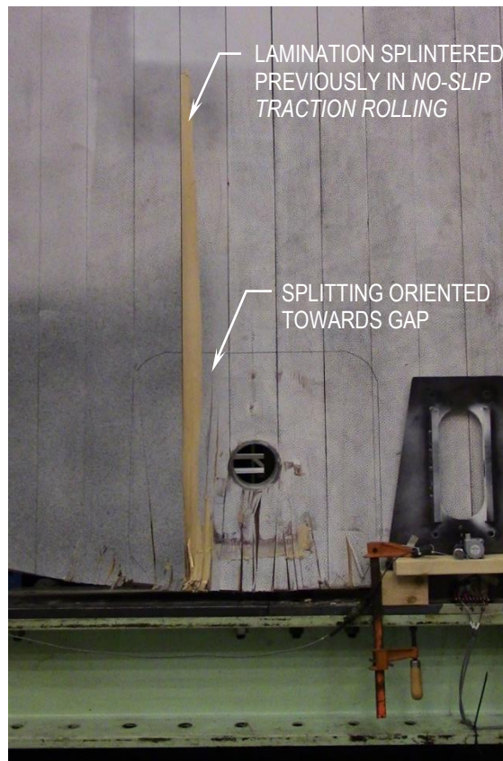
Figure 81. Damage to critical laminations of south elevation of panel ( e = 0.63 ) after Slip-Friction Rocking.
