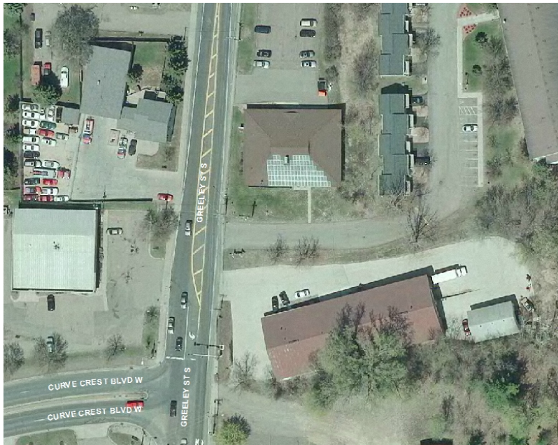
Figure 11 - Greeley Street 2013 Solar Installation
