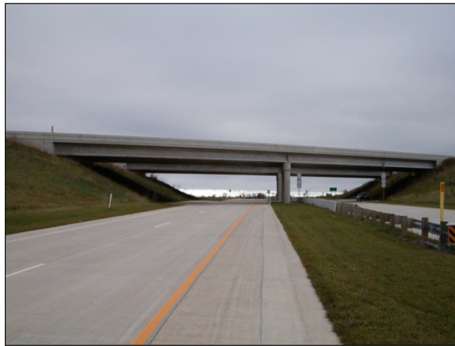
Figure 3.1 Looking North at the Southern Side of B-20-133/134
