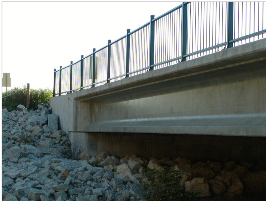
Figure 3.27 (11) North side of East Abutment of B-20-149 Looking SE
