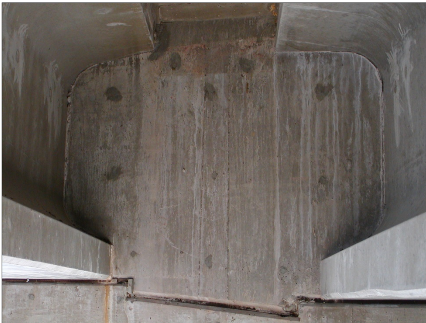
Figure 3.31 (10) West Abutment Between Girders 2 and 3 of B-20-149
