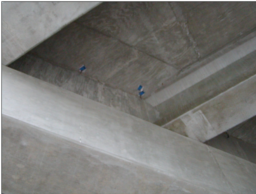
Figure 3.10 (20) Pier Diaphragm Looking West Between Girder 1 and 2, B-20-134
