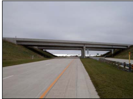
Figure 1.1 South Side of US 151 Overpass bridge, B-20-133
