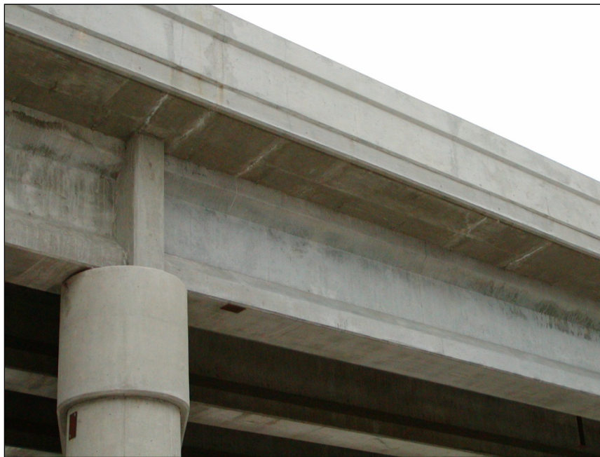
Figure 3.8 (17) East Side of Central Pier on the Southern Side of B-20-134
