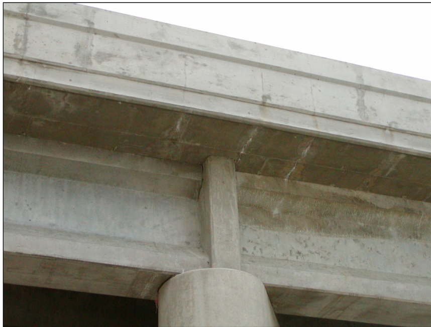
Figure 3.12 (36) Center Pier Exterior on North Side, B-20-134
