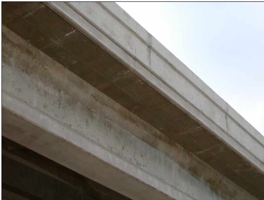
Figure 3.14 (38) West Span B-20-134, North Side
