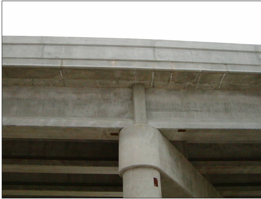
Figure 3.11 (12) North Side Pier B-20-133
