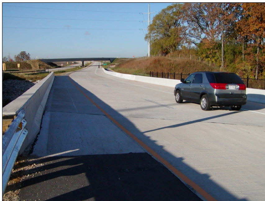
Figure 3.25 (4) Deck of B-20-149 with Traffic Looking West
