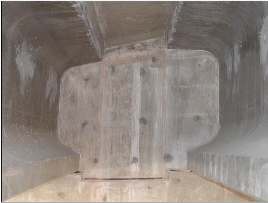
Figure 3.30 (18) East Abutment Between Girders 5 and 6 of B-20-148 Looking East
