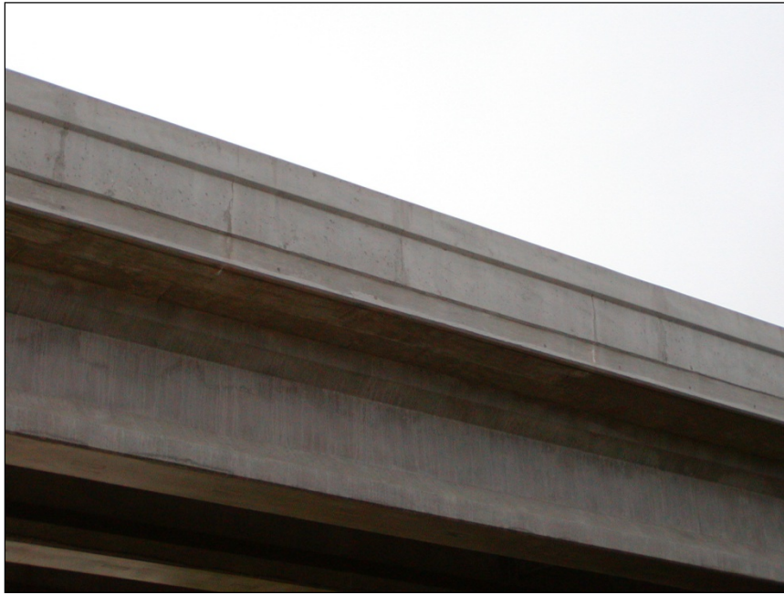
Figure 3.13 (11) West Span B-20-133, North Side
