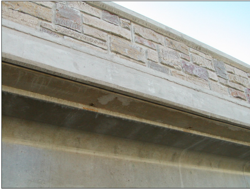
Figure 3.28 (15) Exterior Girder (#7) on North Side of B-20-148 Looking South
