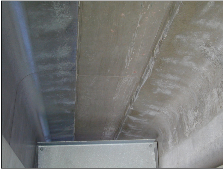
Figure 3.32 (9) 1 st Diaphragm between Girders 1 and 2 on B-20-149
