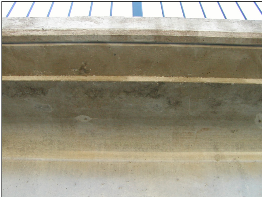
Figure 3.29 (13) Underside of Pedestrian Walkway on North Side of B-20-149
