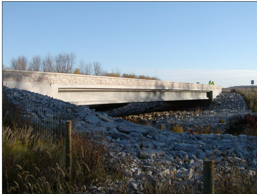
Figure 3.18 (1) B-20-148 South side looking NE
