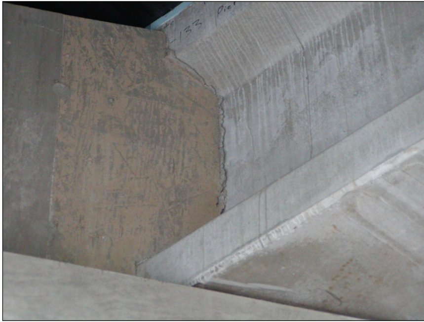
Figure 3.9 (4) Interior Diaphragm of B-20-133 Above Pier, at Girder 2 Looking West
