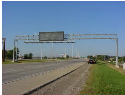
Figure 3.8: Sign Bridge S-40-404 Located on the “Airport Spur” in Milwaukee.
