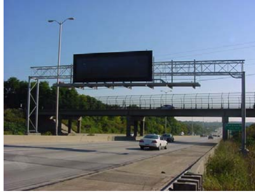
Figure 3.7: Sign Bridge S-67-402 Located in Waukesha County over Eastbound IH 94.
