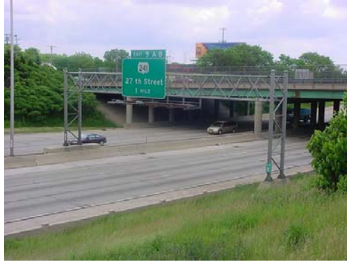
Figure 3.1: Four-Chord Pipe Truss Configuration used by WisDOT.
