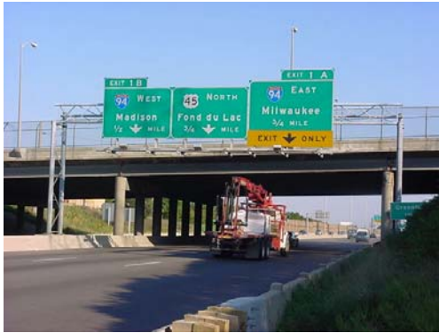
Figure 3.9: Sign Bridge S-40-156 Over IH 894 in Milwaukee, County.
