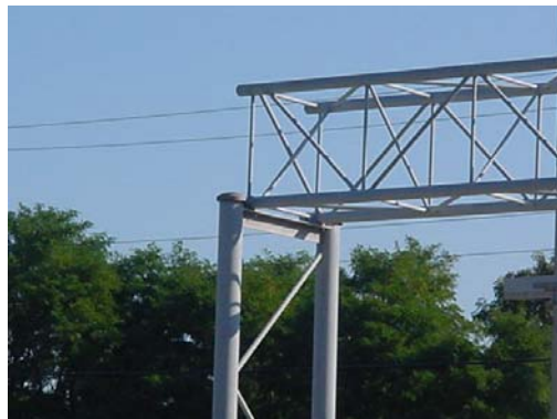
Figure 3.3: WT Support Strut used in WisDOT Sign Support Structures
