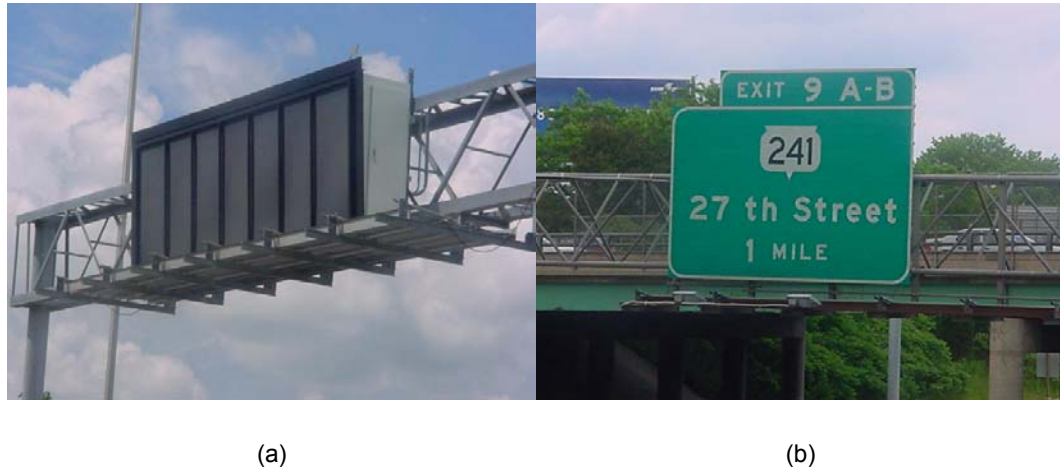
Figure 3.6: Sign Types used in Wisconsin: (a) Variable Message Sign (VMS); (b) Type I Aluminum Printed Sign.
