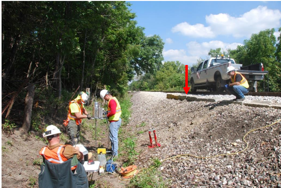
Figure 16: Concrete site view. Note ditch location. V-blocks are highlighted by red arrow.
