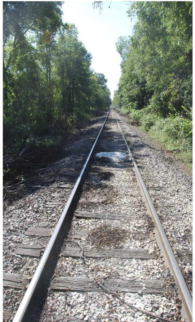
Figure 6: Ballast site track condition
