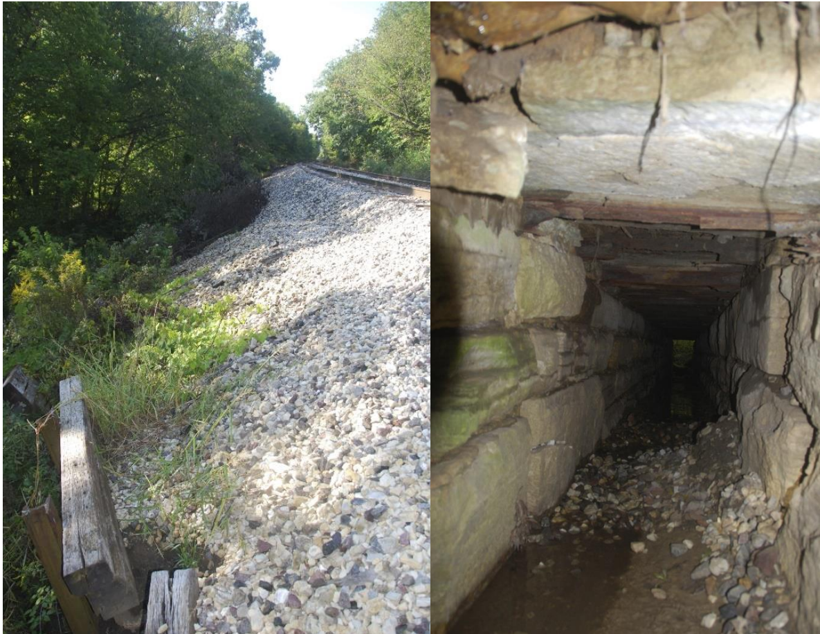
Figure 21: View of the culvert section.
