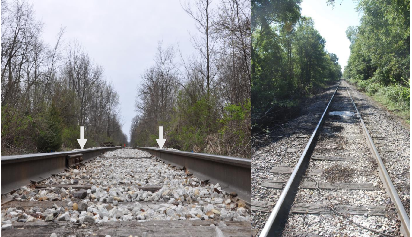
Figure 46: Subgrade failure
