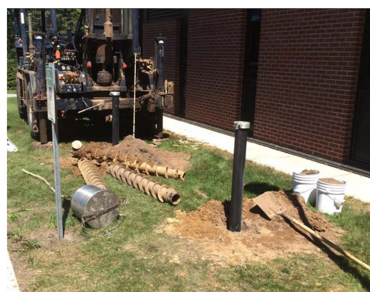
Fig 3. Summer 2018 551 well drilling
