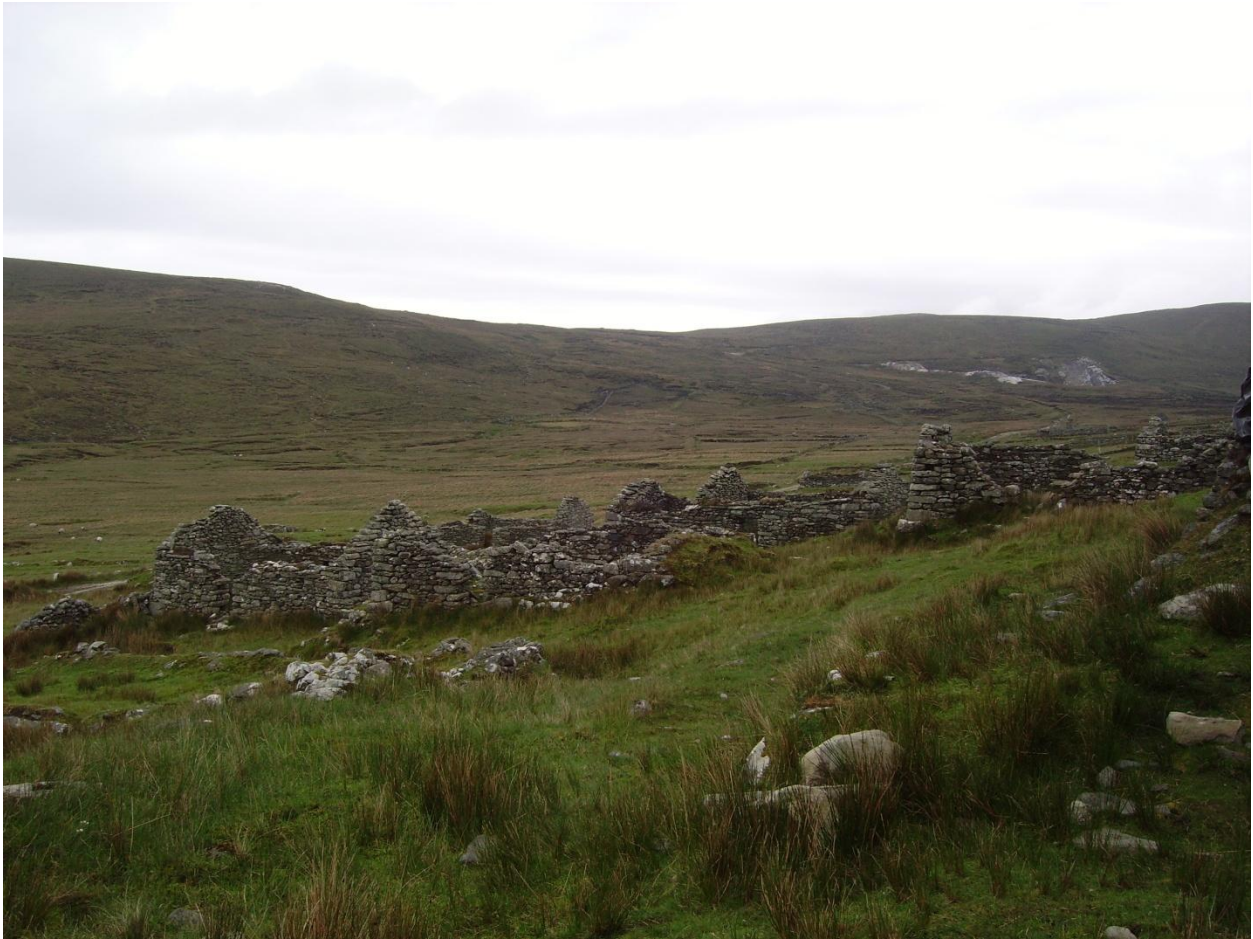
Figure 3. Houses in various states of ruin.
