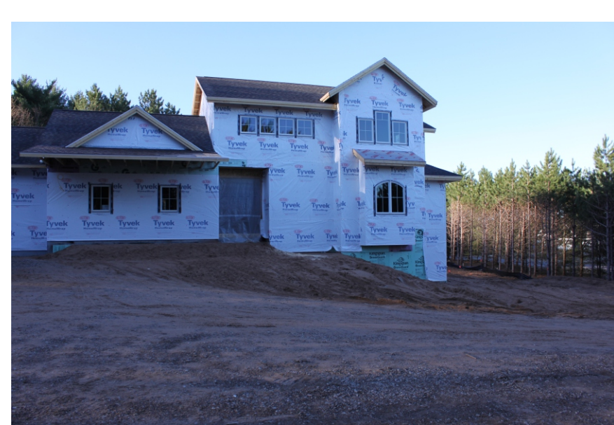
Fig 6. Typical Huntsinger Heights septic system absorption field. This newly constructed absorption field is located in the glacial outwash on the south side of lot 19 (Fig. 7)
