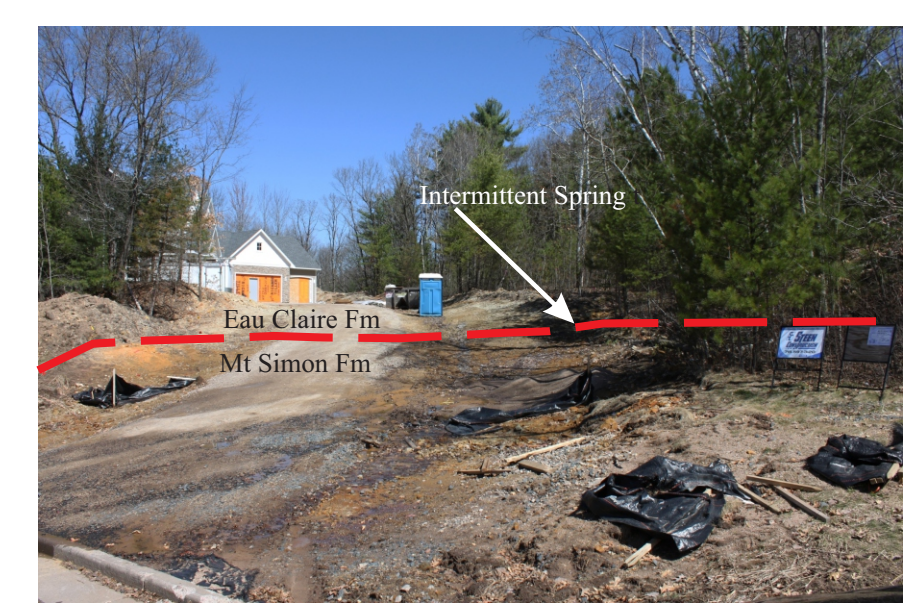
Fig 2. Home construction (Lot 15) built directly into bedrock at the Mt Simon and Eau Claire Fm. contact. An intermittent spring at the contact illustrates horizontal fracture flow in this hydrogeologic system.
