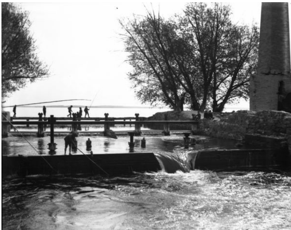
Fig 2- Yahara River Dam- Outlet of the Yahara River. The ruins of the original Farwell Mill are on the right, suggesting this photo was taken before the city constricted a new dam, and after the original mill burnt down in the 1890s. Note the drop of water and the scale of the child. This suggests the dam had a head of about 3 or 3.5 feet.
