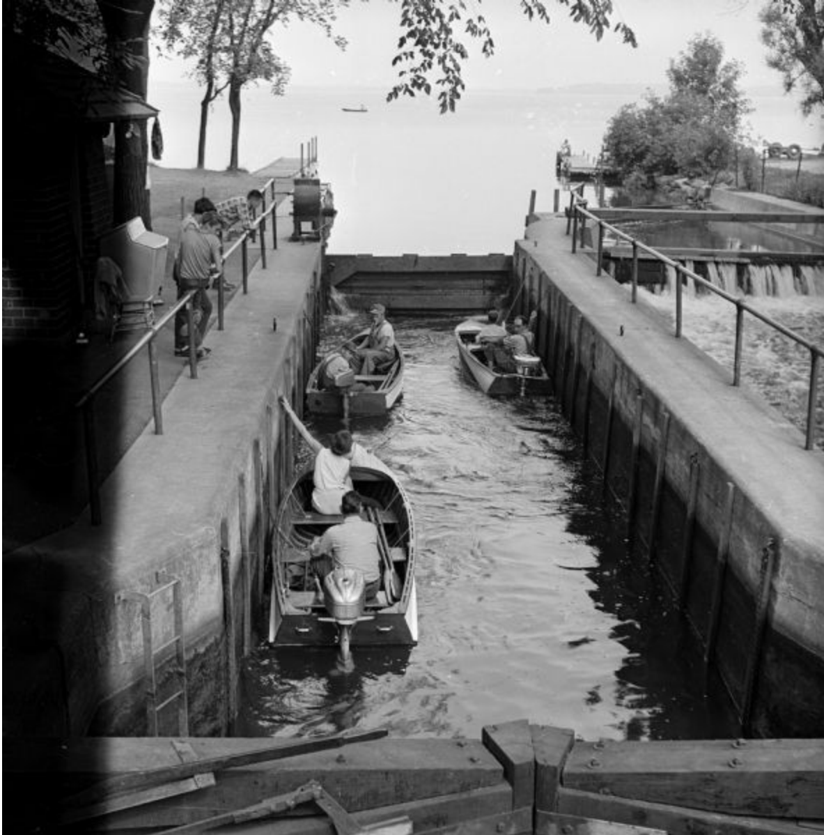
Fig 4- Original Tenney Park Lock and Dam in the early 1950s. Judging by the water line and the boaters, we estimate the dam to have about a 4 foot head, which is in agreeance with the water level orders placed in 1931 Wisconsin Historical Society, Arthur M Vinje, Summer Scenes at Madison Parks and Beaches, Image ID: 108797. Viewed online at https://www.wisconsinhistory.org/Records/Image/IM108797
