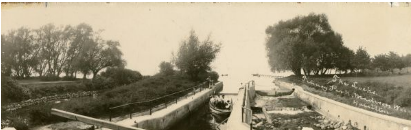
Fig 3 - Image of the original Tenney Park Lock and Dam in 1906. Again, judging by the scale of people and the drop of water, the head of the dam is around 3-4 feet.
