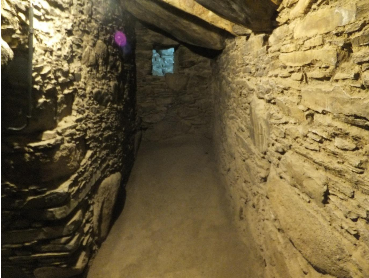
Figure 2.13. Image inside third floor of Chullpa in Willcawain. Note the slanted roof.
