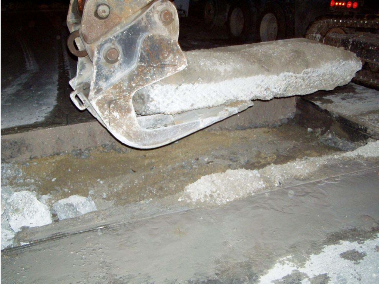
Figure 4. Slab Crab bucket removing damaged concrete in repair area.
