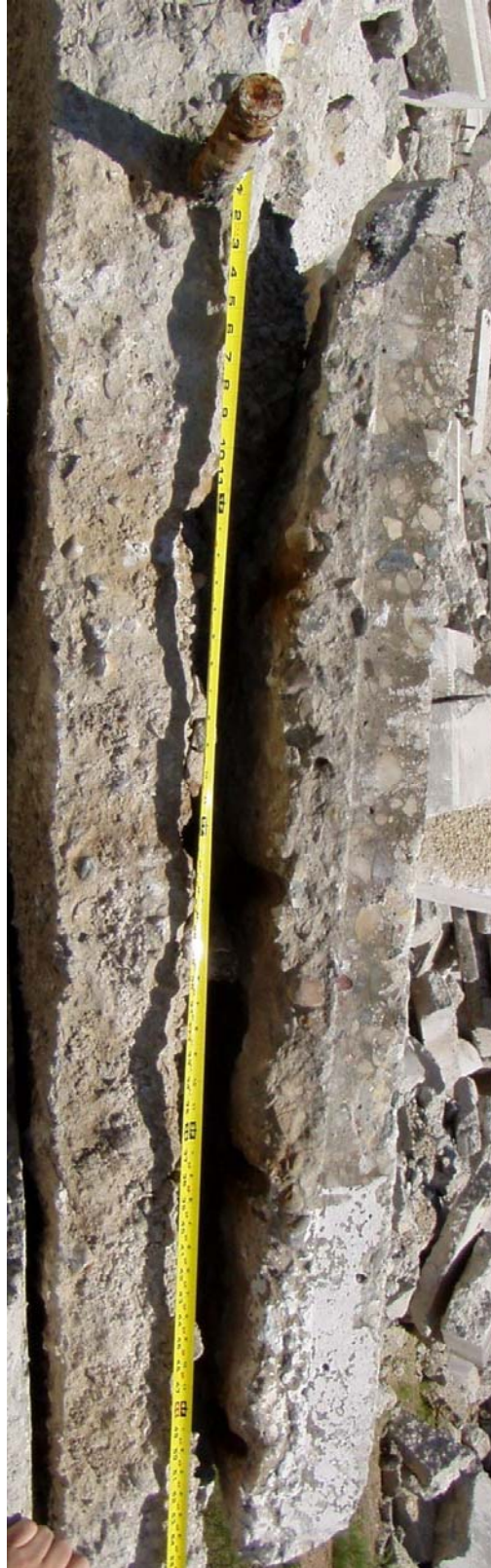
Figure 11 Mid-depth delamination of slab extended from corner (bottom of photo) to approximately 5 ft. from edge (top of photo), before appearing as surface crack.
