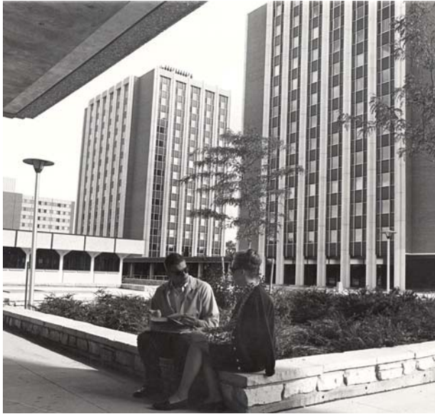
Figure 16: Ogg Hall, 1960's. Lenburg, Norman. Ogg Hall . ca. 1960-1969. Photograph. University of Wisconsin Madison Digital Collections, accessed November 15, 2012.
