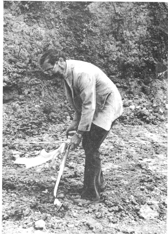
Ed Rowe presenting the ceremonial shovel to Ragnar Rollefson (left) and taking a shovelful of soil himself (above). They are at bedrock level of the 8 ft. excavation for Aladdin.
