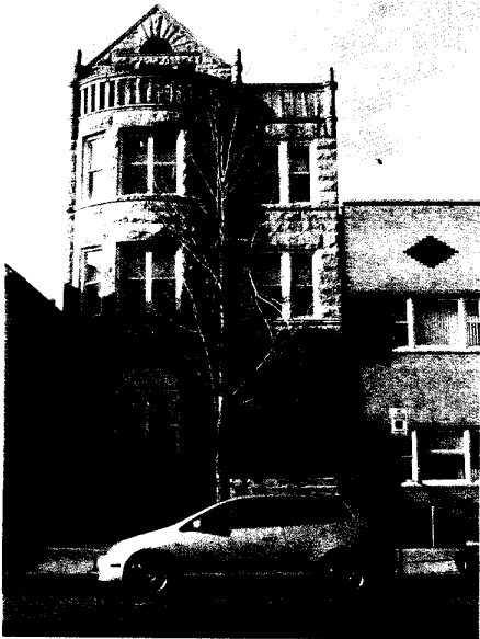
Figure 3.14: A residential building in the Romanesque Revival Style at 266 West 24 th Street. Source: photograph by Chuo Li, 2004.
