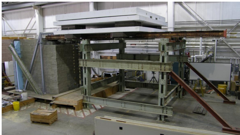
Figure 4-4: Completed GRS abutment
