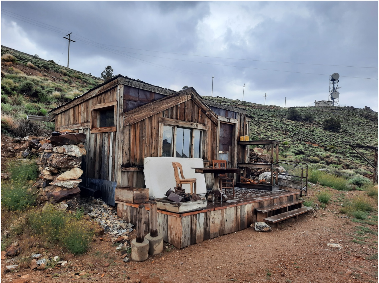
Figure 29: Building at Cerro Gordo.
