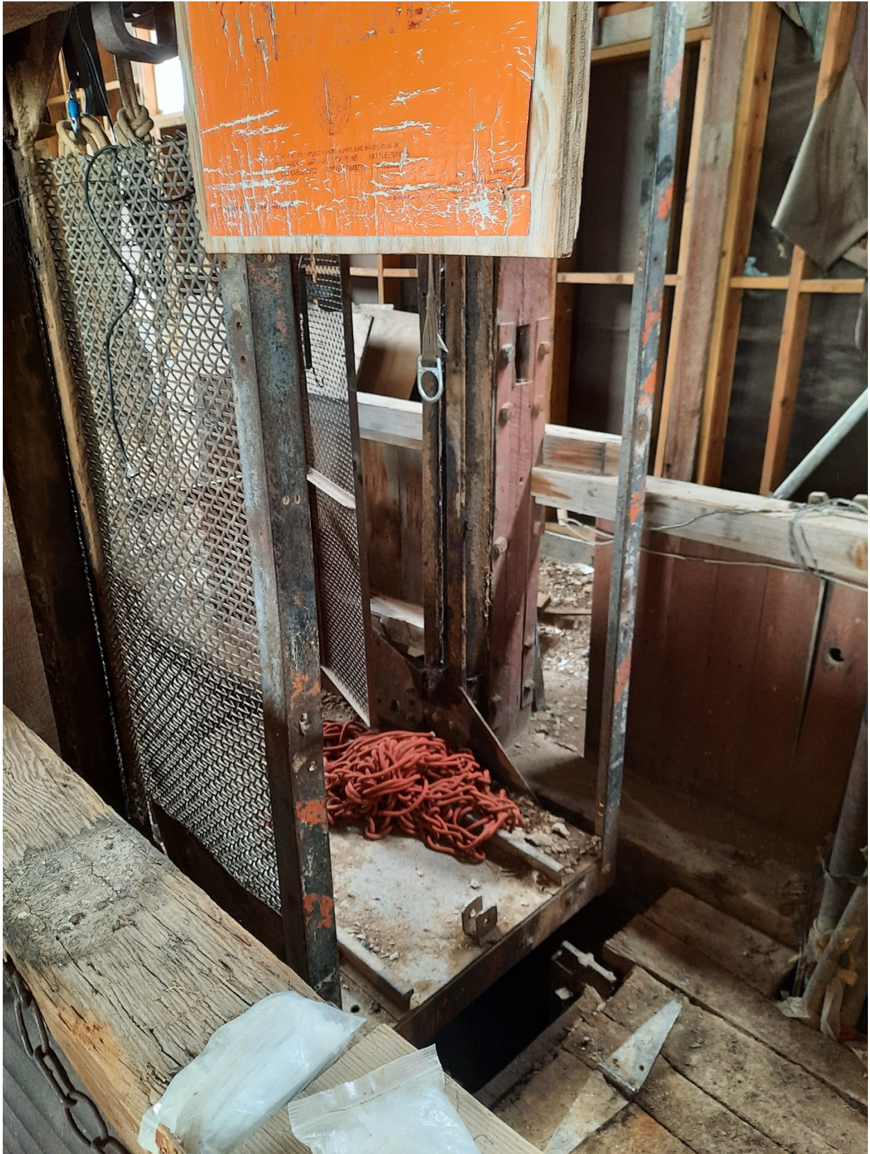
Figure 52: Cage to enter the mines.
