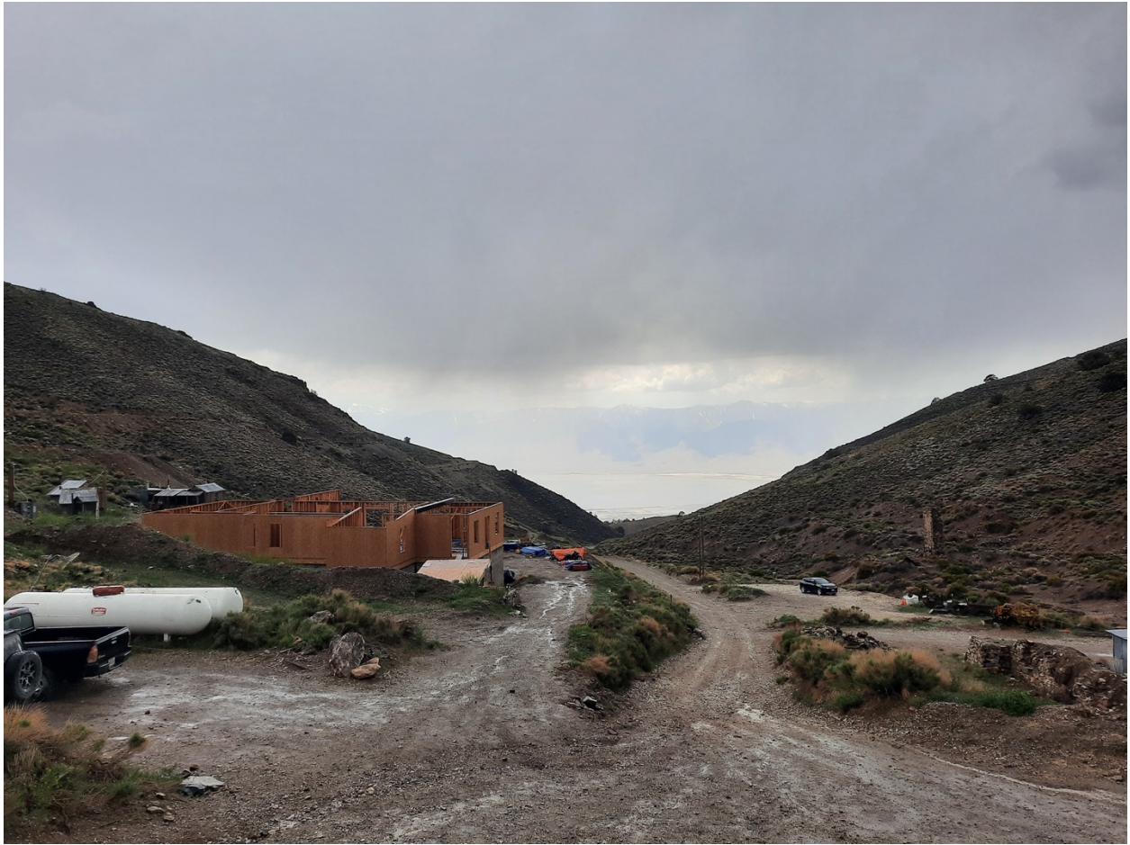
Figure 16: American Hotel rebuilding site.
