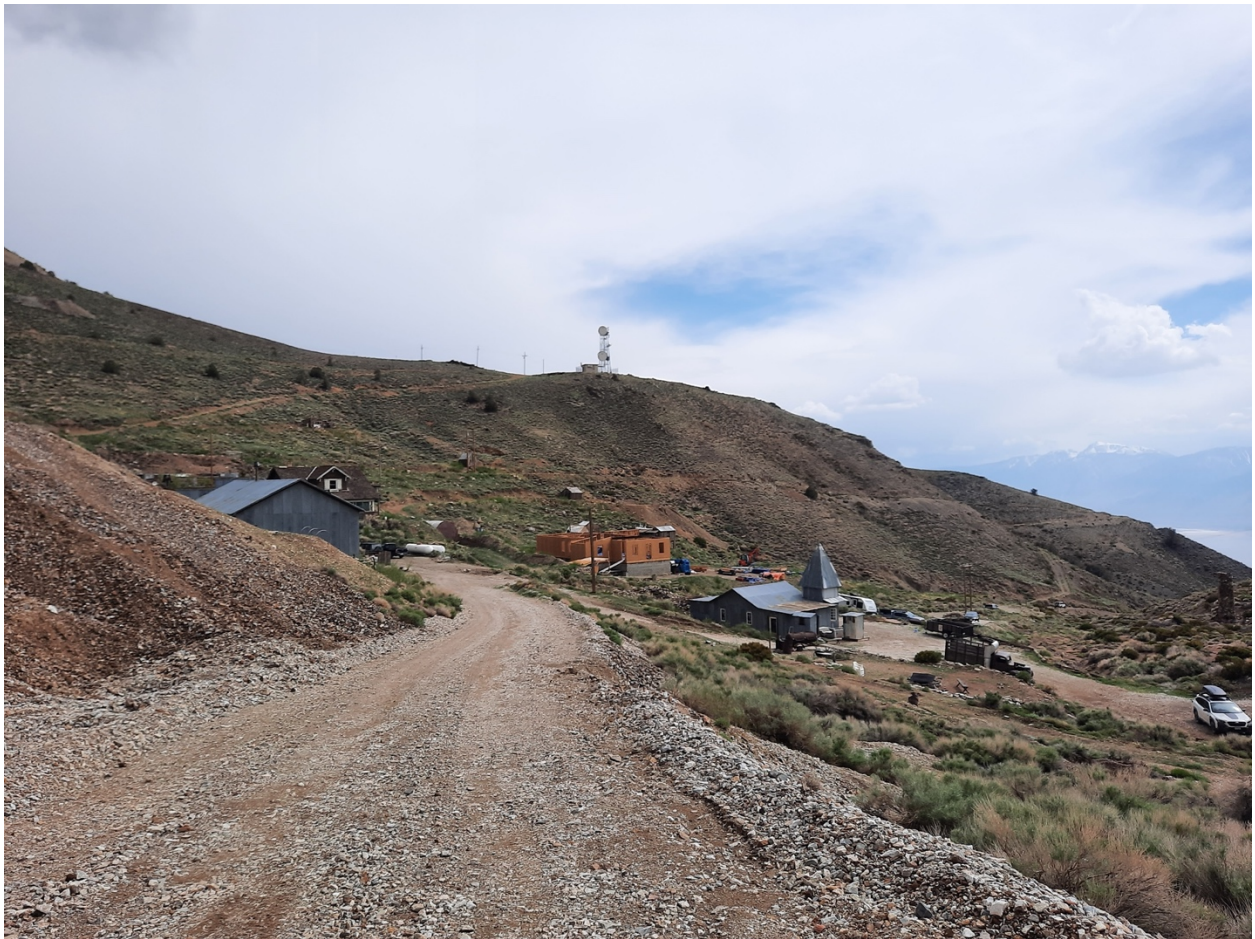
Figure 46: Road from the Hoist House.
