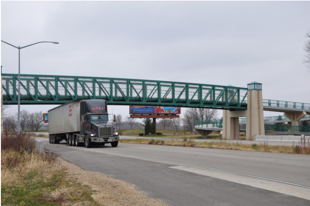
Figure F) Footbridge over Highway 30 in Madison.
