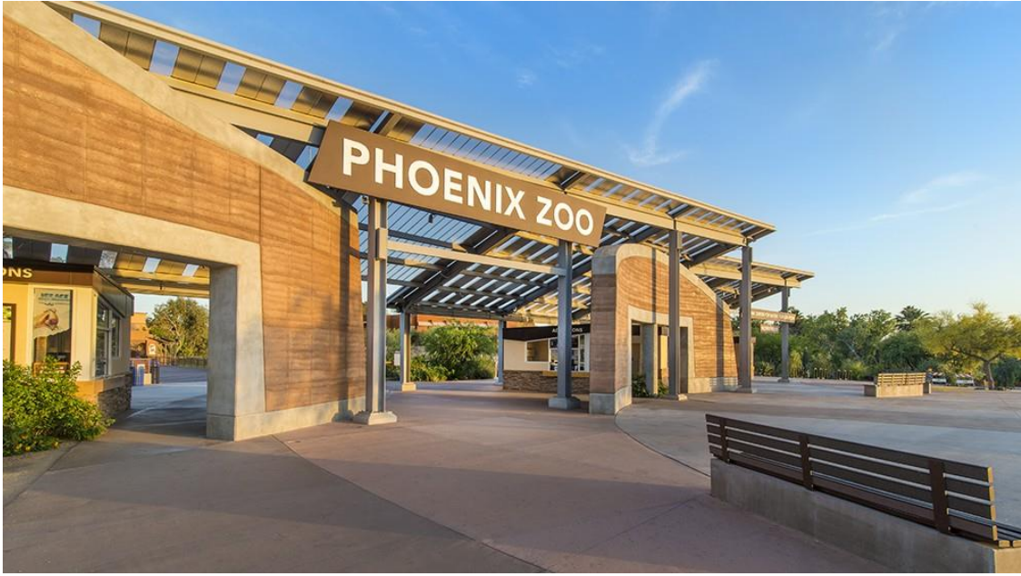
Figure 2 photo of Phoenix Zoo entrance that was made of rammed earth [Source: wdm Architects]
