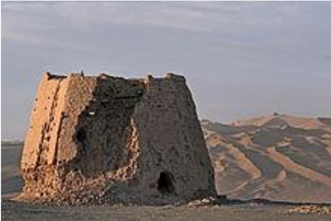
Figure 1: The ruins of a Han dynasty (202 BCE – 220 CE) Chinese watchtower made of rammed earth at Dunhuang ( Source weikipedia )
