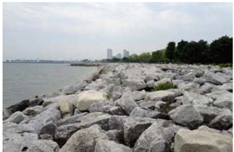
These large boulders were placed at the south end of Bradford Beach and help to mark the end of the beach as well as prevent erosion.
