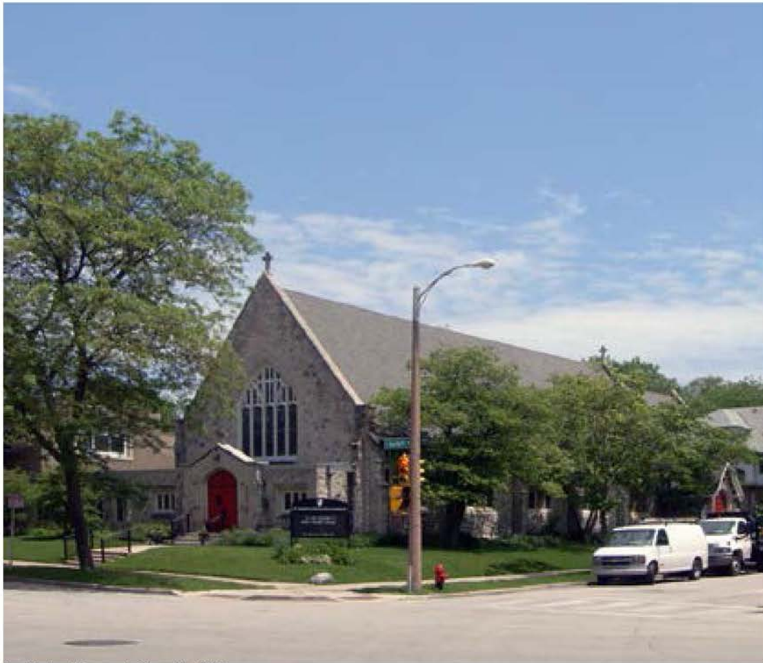
St. Marks Episcopal Church, 2013.
