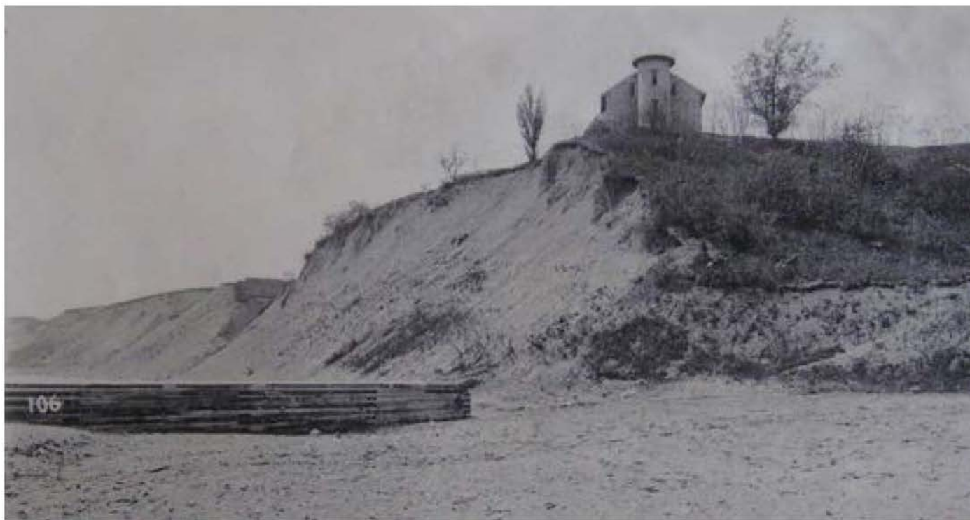
The the erosion of the bluff. near the 1854 North Point Lighthouse.
