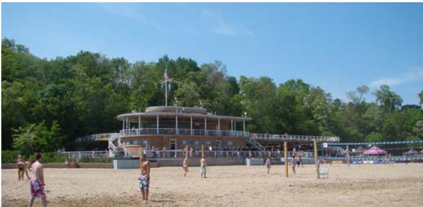
View of the Bradford Beach Bath House from the beach (looking North).
