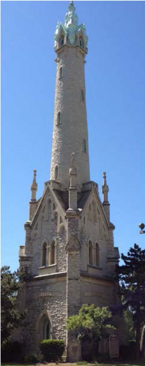
The Historic Water Tower, built in 1873, after which the surrounding neighborhood is named.
