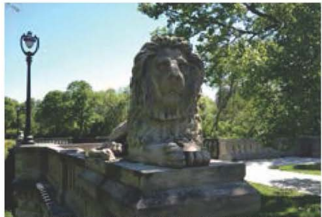
Detail of a lion on the Lion Bridge, after undergoing restoration.
