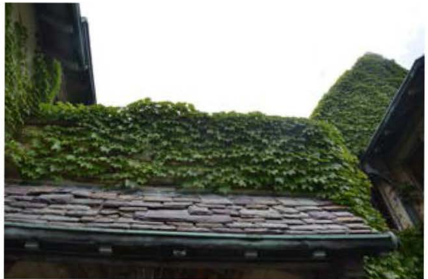
Roof detail showing tiles.
