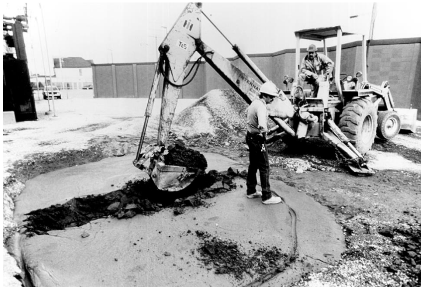
Figure 2.2: Excavating CLSM with backhoe (ACI 229R, 1999).
