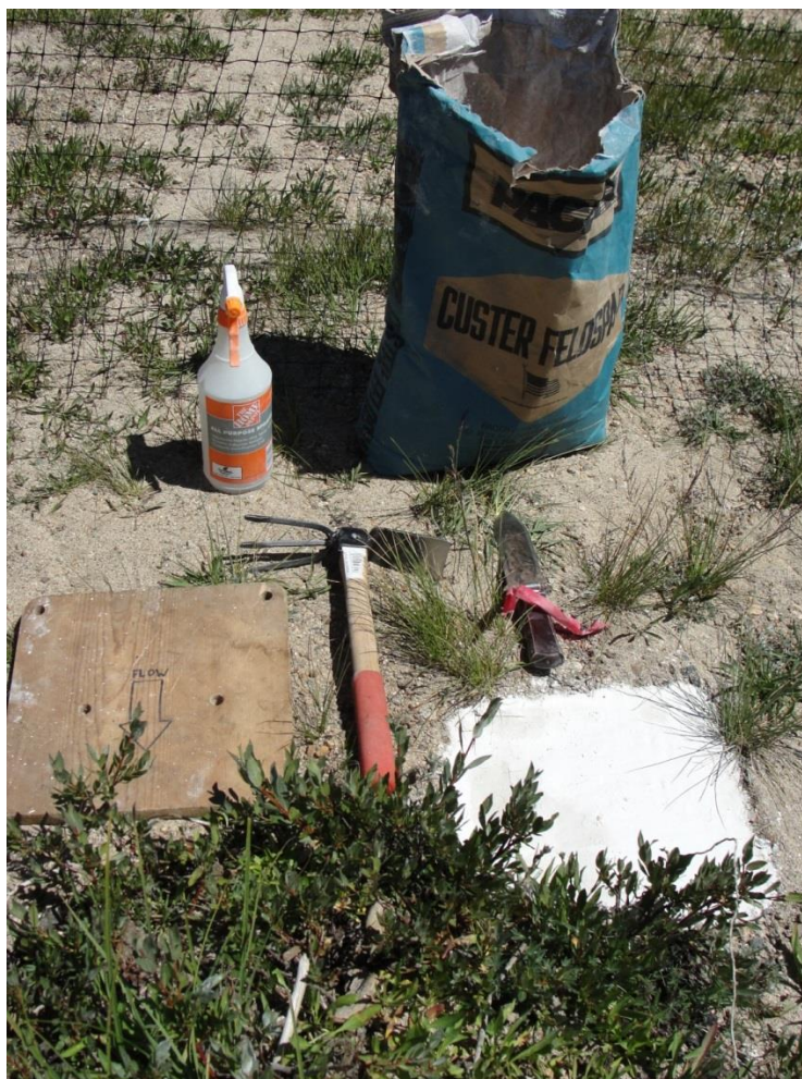
Figure 1: The material required to install a clay pad are (clockwise from the top): white powder feldspar clay, digging tools, and a pad template, and a spray bottle. In this image, recently installed clay pad is visible on the upstream side of a willow.
