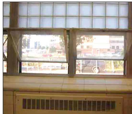
The only cooling system in the Dairy plant and short course cheesemakers all know how well it works on a hot summer day.
